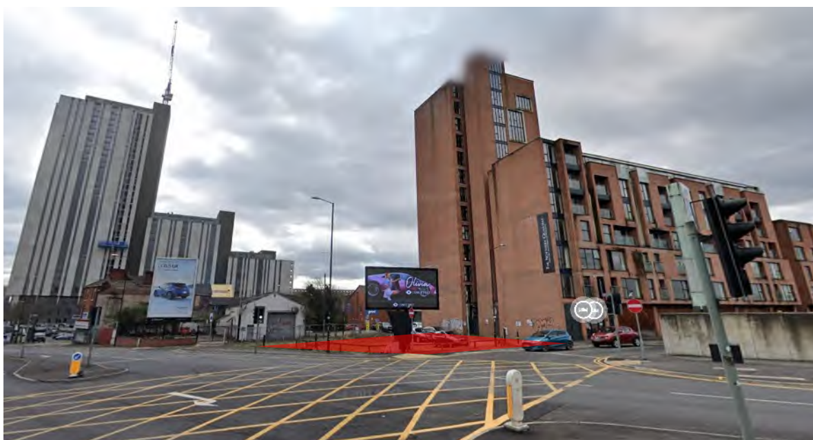
Figure 1: Looking south towards the cleared plot which forms the Site, with Great Ancoats Street (left) and Laystall Street (right)
