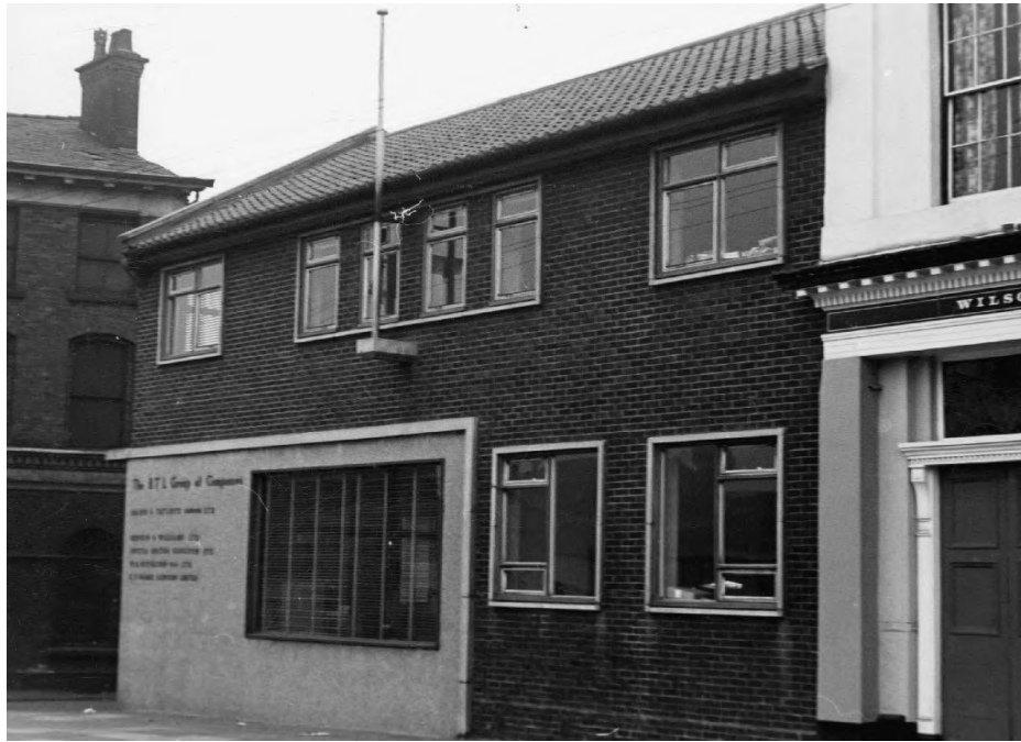
Figure 15 – The adjacent 1950s commercial building to the south of the White House on Great Ancoats Street in 1967. (Source: Manchester Archives)
