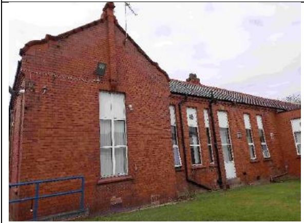
Photograph 15: Eastern elevation of B4
