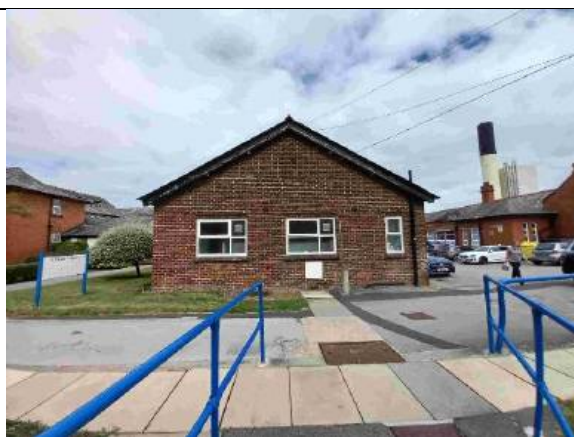
Photograph 20: Southern elevation of B5a
