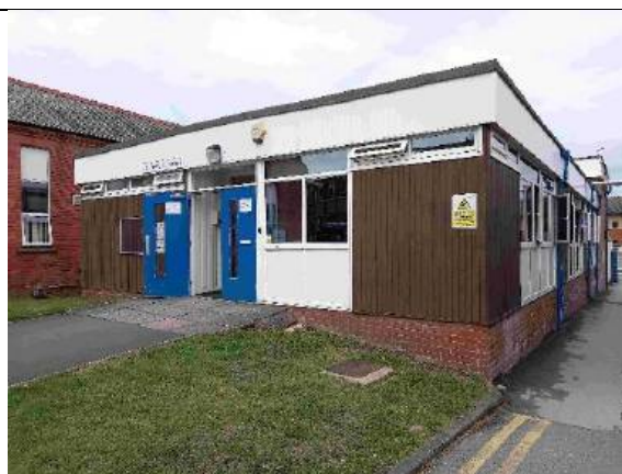
Photograph 10: Southern elevation of B3
