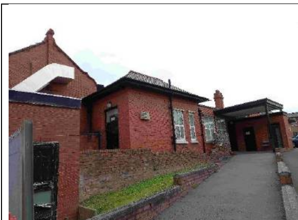
Photograph 17: Western elevation of B4
