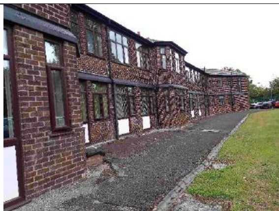
Photograph 6: Southern elevation of B2
