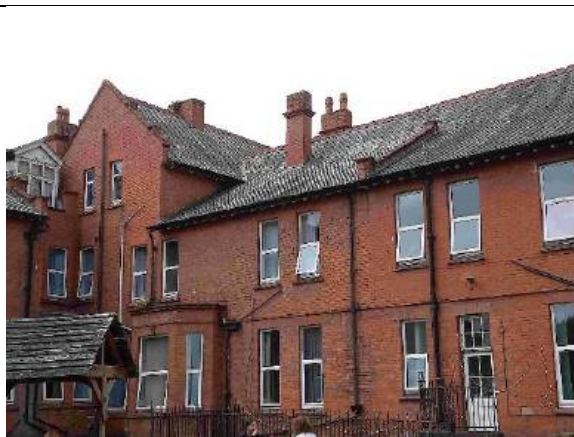
Photograph 22: Eastern elevation of B5b
