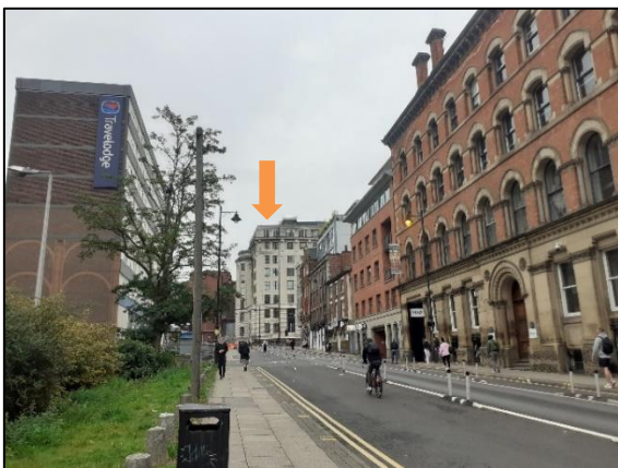
Figure 3: View looking east along Blackfriars Street. The approximate location of the roof terrace is indicated.
