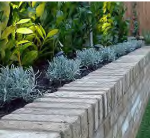
Brick planter/brick walls defining private thresholds
