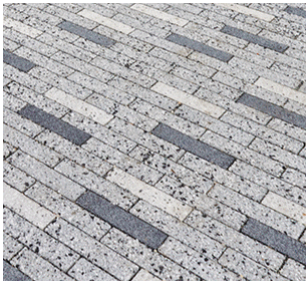
High quality exposed aggregate concrete block paving
