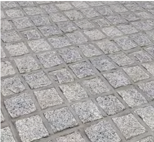
Sett paved crossover
