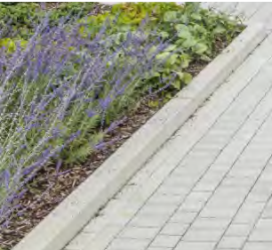
Exposed aggregate kerb upstands to planting areas
