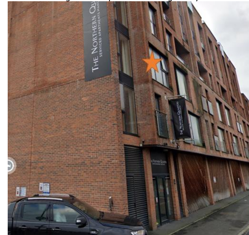
Figure 13: Monitoring Location at existing services apartment building on Laystall Street next to proposed hotel
