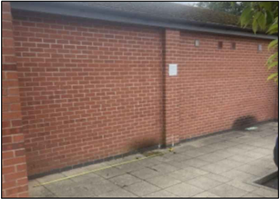
PHOTOGRAPH OF EXISTING ELEVATION A
