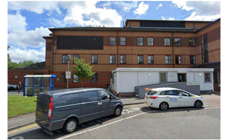
02. FRONT FACADE FROM CRUMPSALL WAY
