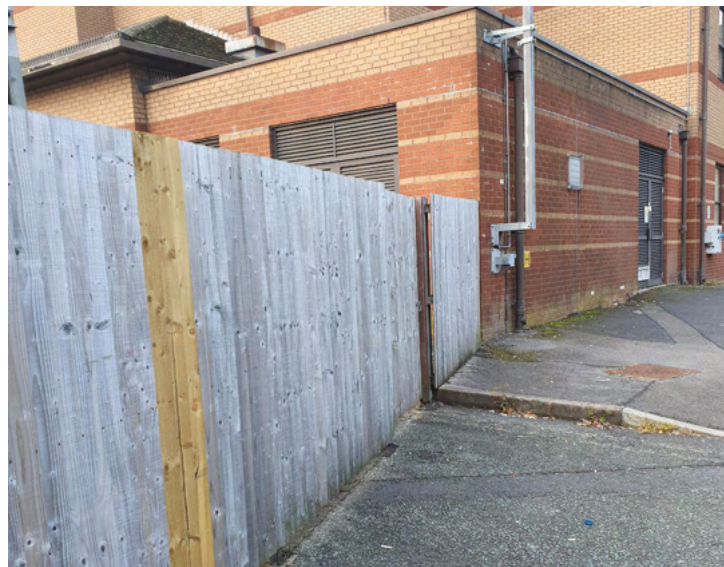
05. VIEW OF EXISTING SUB STATION
