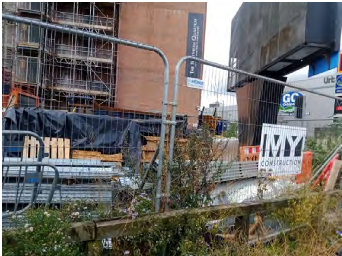
Photograph 2: View looking southwest showing skips as well as piles of metal and wood stored on site.
