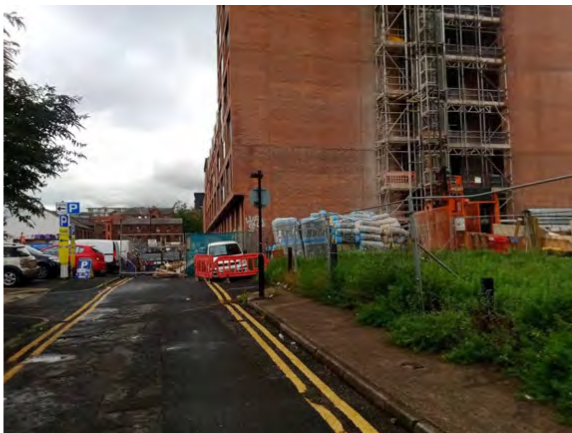
Photograph 4: View looking west along Lomax Street, showing storage of insulation and other construction materials.
