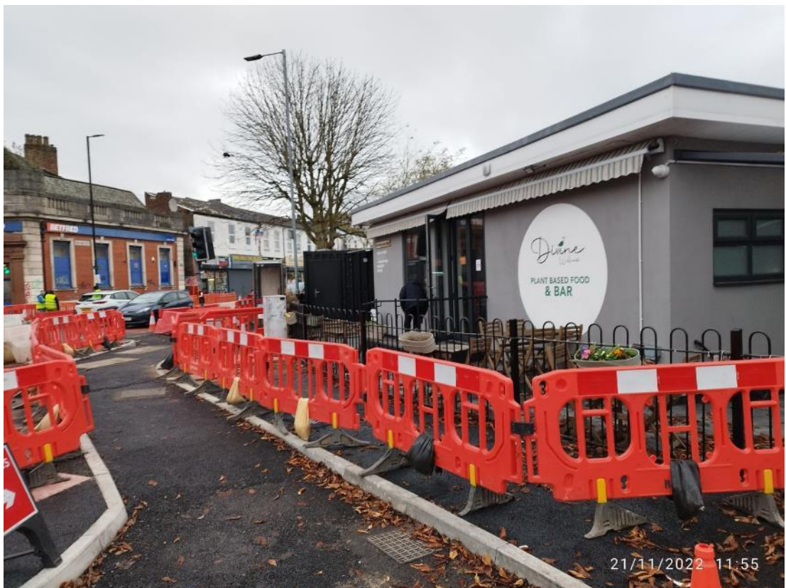
(Figure 4 – Photograph showing the frontage of the café / restaurant and the CYCLOPS highway junction scheme works that are taking place directly outside)
