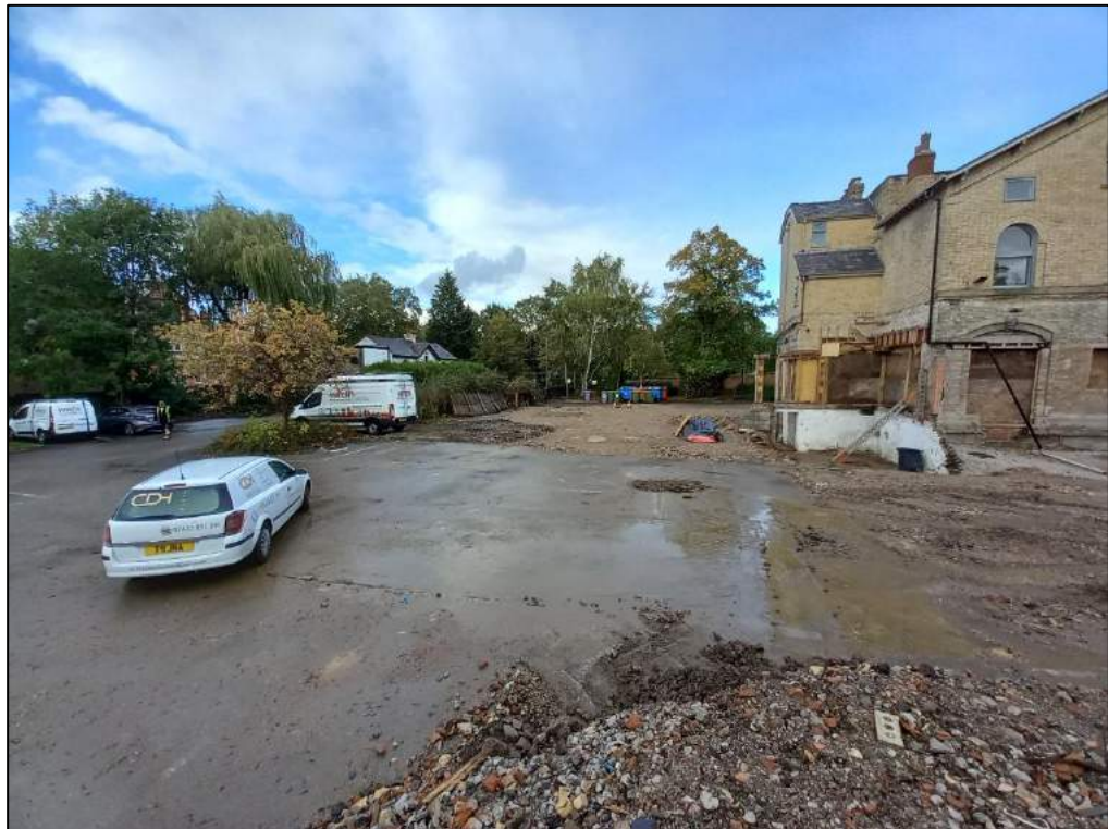
Photograph 03: Looking north, showing partially demolished former The Greenfinch building. October 2022
