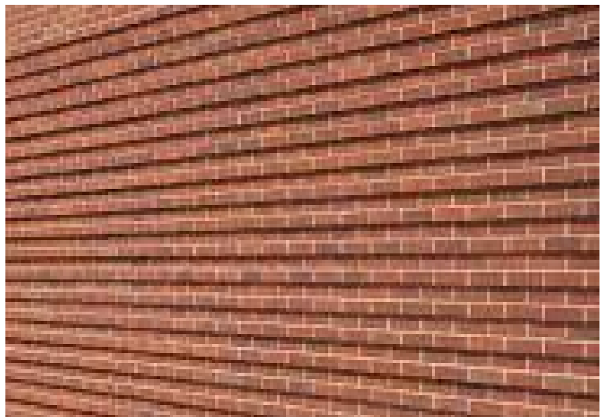
Red Brickwork Detailing
