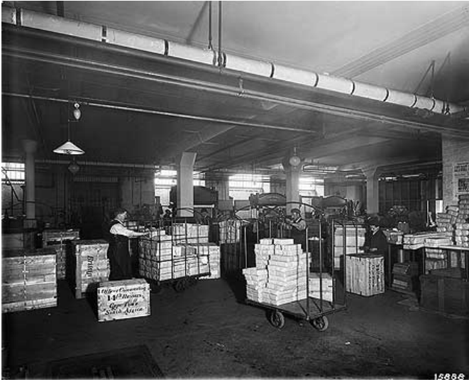
Image 4: The basement of Churchgate House, taken in 1900 (Historic England archives).
