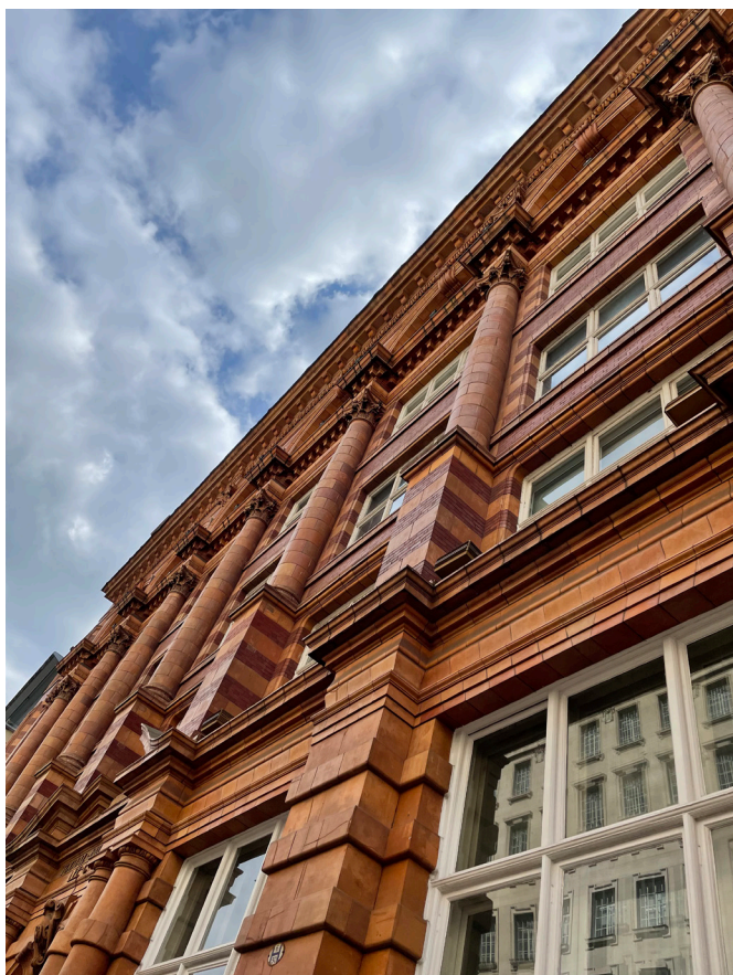
Image 10: Detail to Oxford Street facade.
