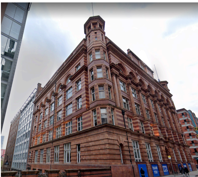
Image 01: 56 Oxford Street, Oxford Street and canal side elevations.
