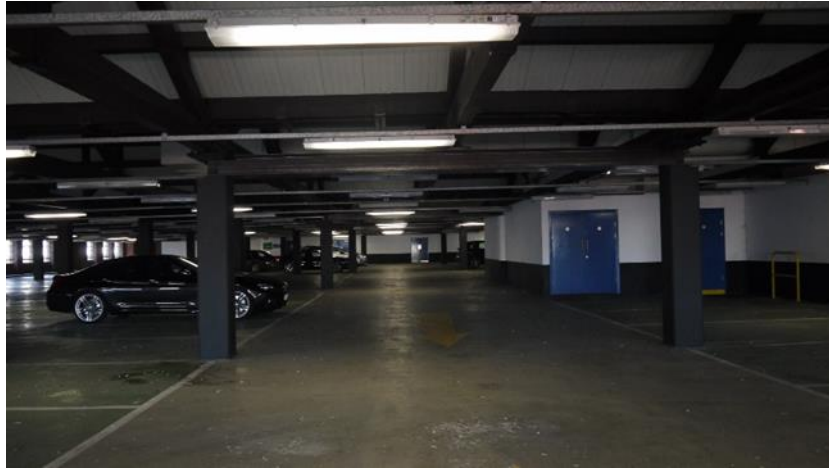
Figure 4.1: Column removal & installation of transfer beams
