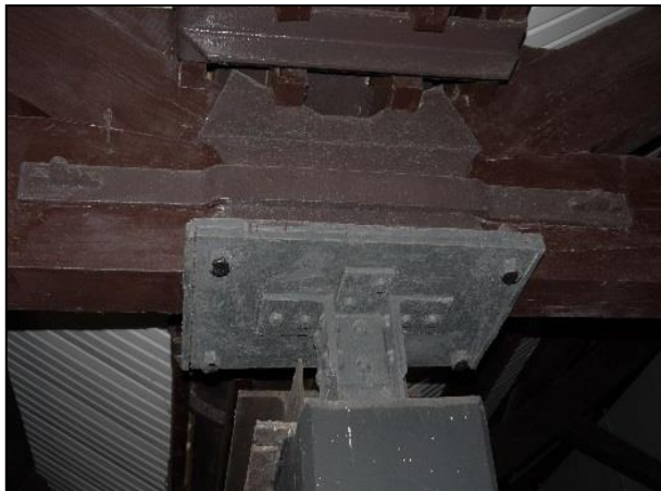
Figure 4.2: Column head detail supporting roof truss
