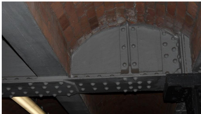
Figure 6.2: Web stiffeners / angle connection
