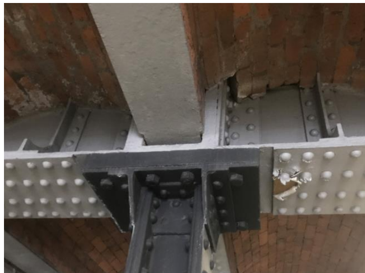
Figure 6.1: Connection junction at floor
