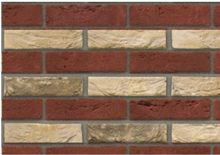
Banded Brickwork - Red / Buff
