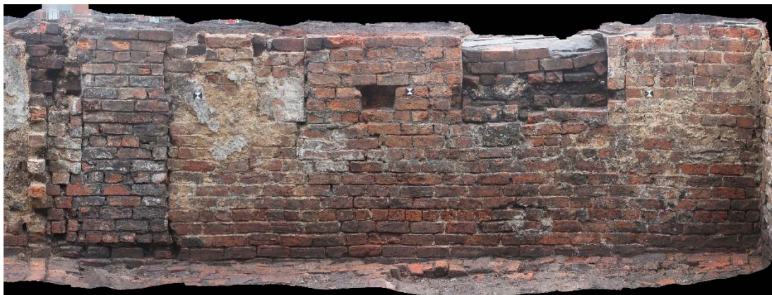
Plate 72: The north-west-facing elevation of C3 , with the surviving Phase 1 cellar light and door (later blocked)
