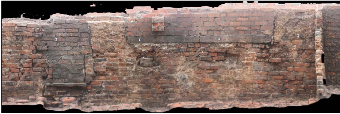
Plate 68: North-west-facing elevation of C9 , with the surviving Phase 1 cellar light and door (both later blocked)
