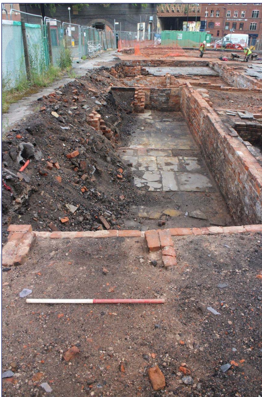
Plate 27: C1-3 , looking north, with a blocked doorway visible on the northern elevation of C3
