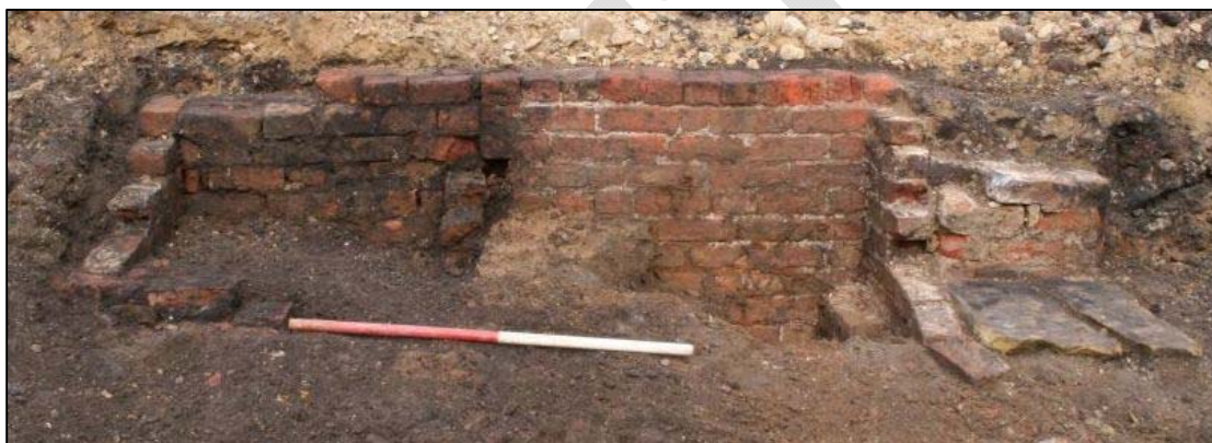
Plate 53: Blocked cellar light, R10 , looking north-west
