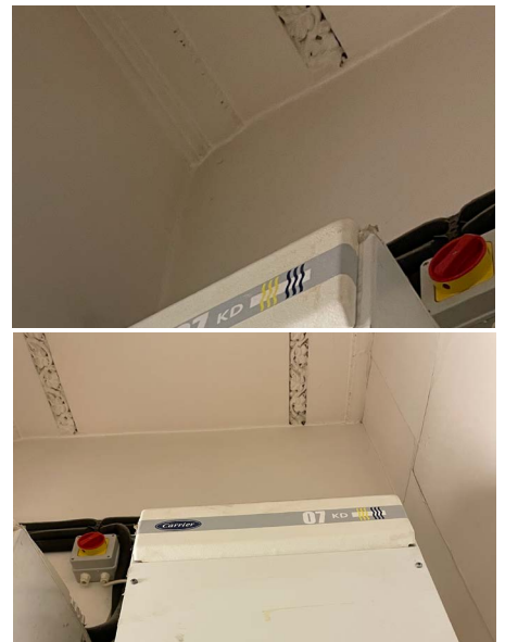
Ceiling details within rear area of unit - to remain untouched
