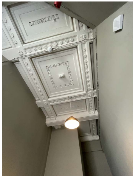
Ceiling details in rear communal staircase
