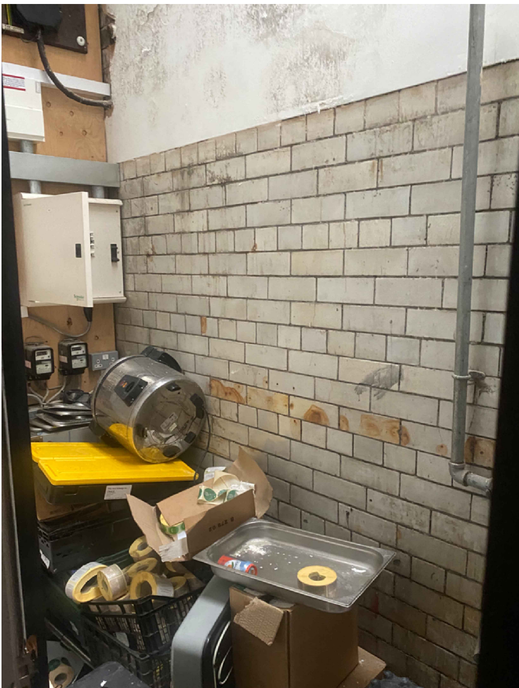
EXISTING BASEMENT BACK OF HOUSE
