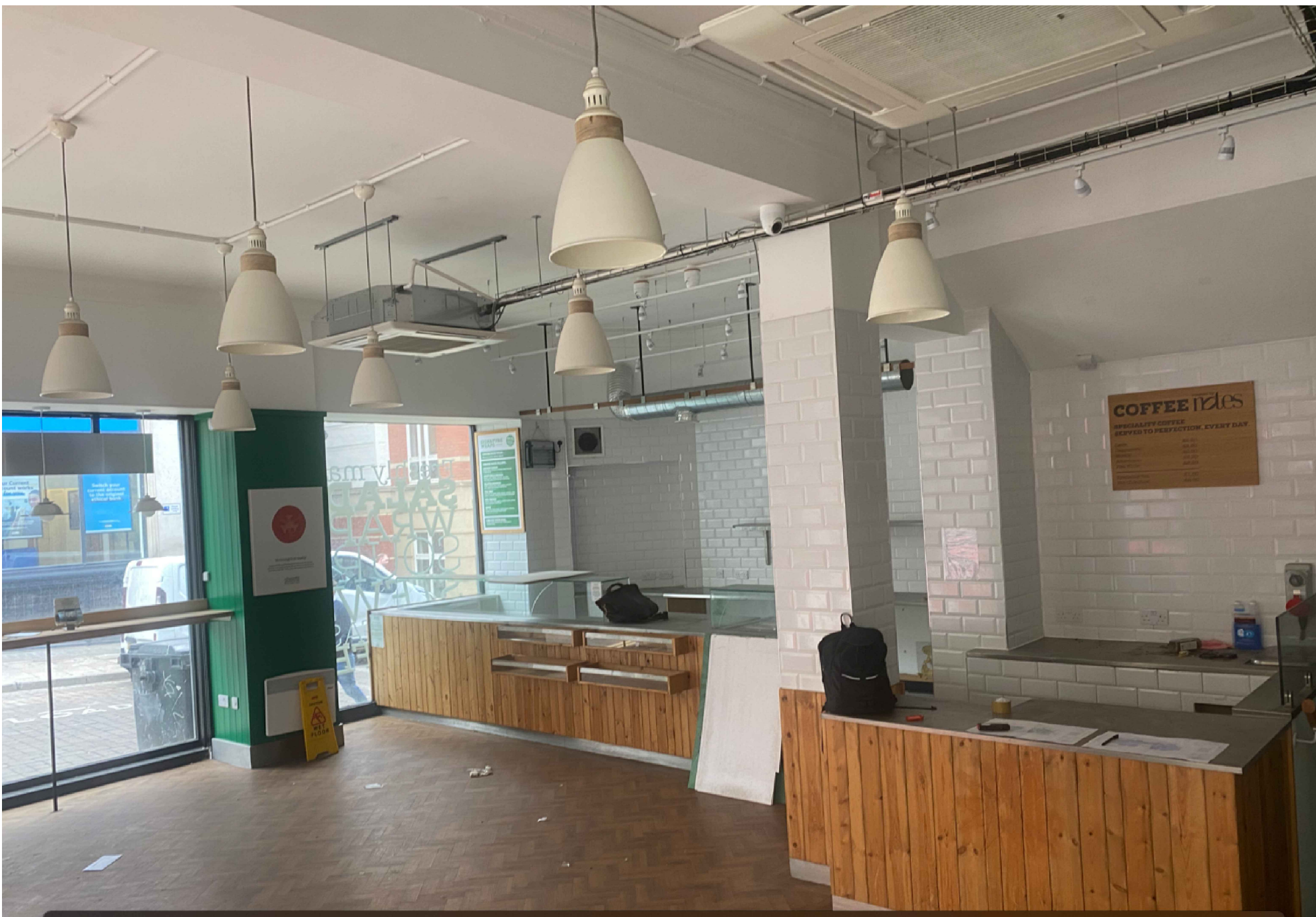
EXISTING GROUND FLOOR SERVERY AREA
