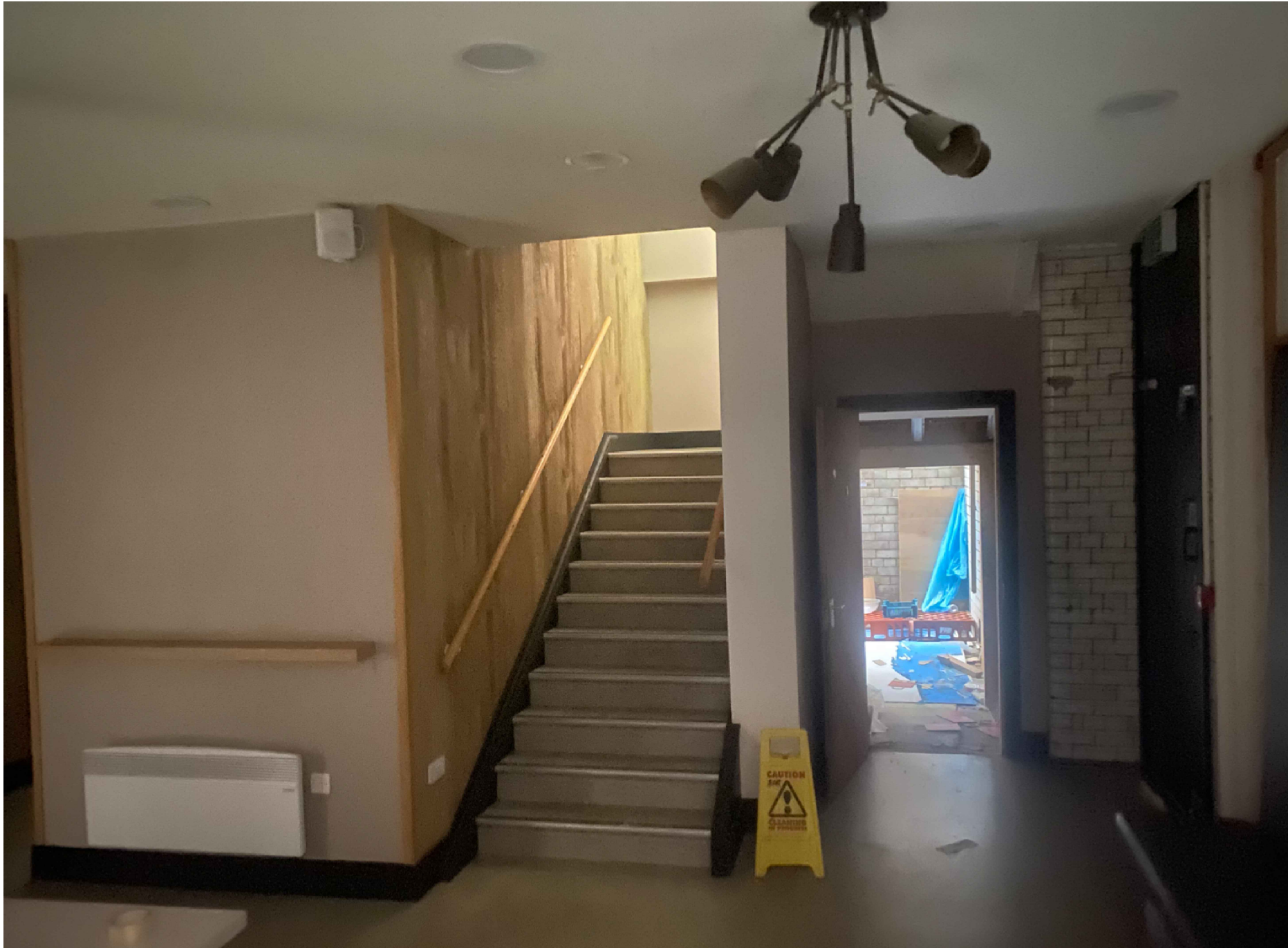
EXISTING STAIRCASE FROM GROUND FLOOR
