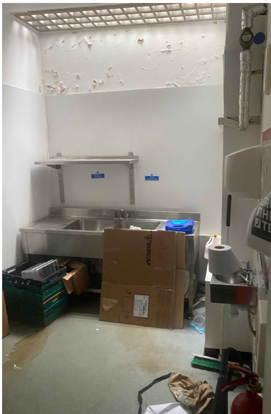
EXISTING BASEMENT BACK OF HOUSE
