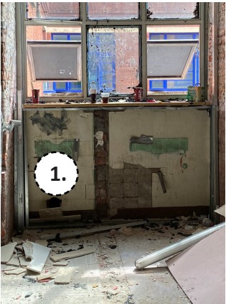
1. Existing South East Wall
