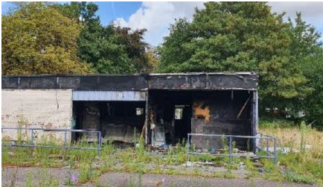
Images illustrating examples of the current condition of existing buildings on site
