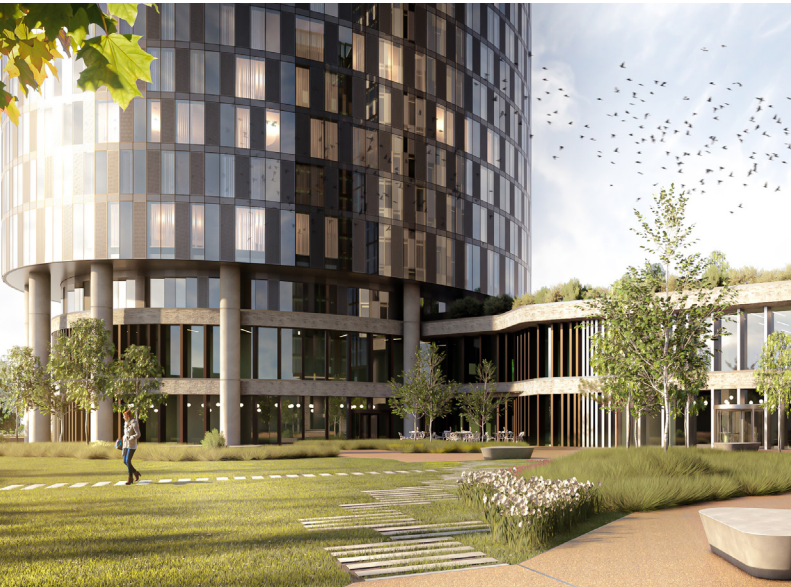
Crown Street Phase 2 Brick bands at level 01 and 02
