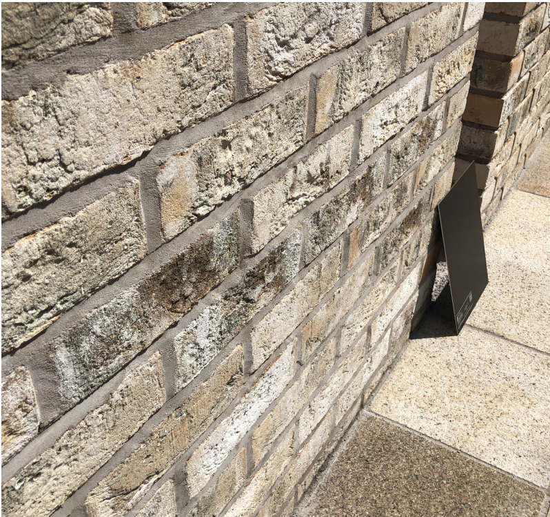
Crown Street Phase 1 - Sample Panel Indicative brickwork, mortar and pointing only Photographed 13.05.20
