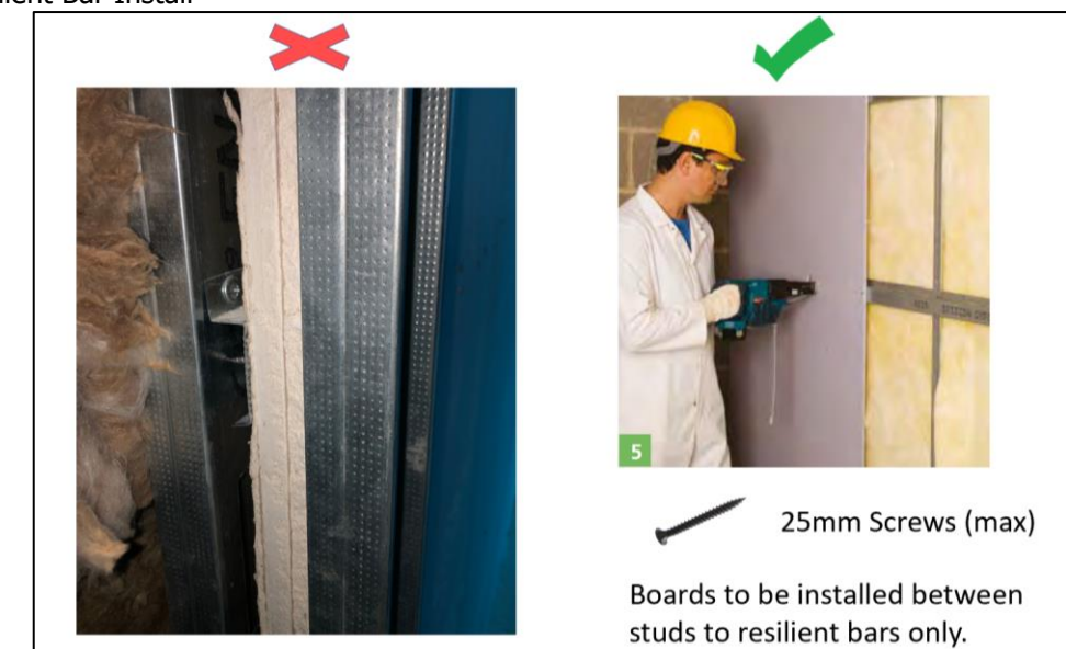
Figure 12: Resilient Bar Install
