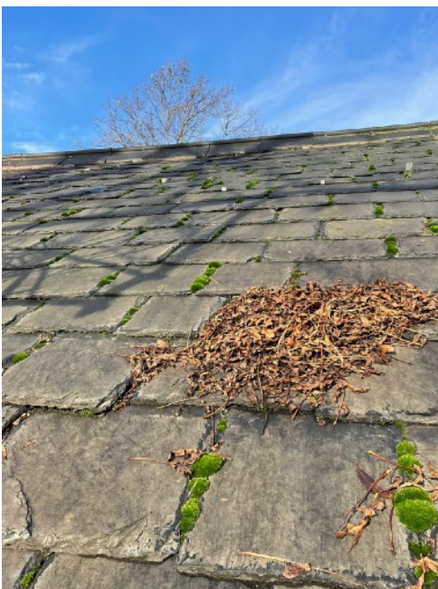
Existing slates on rear elevation
