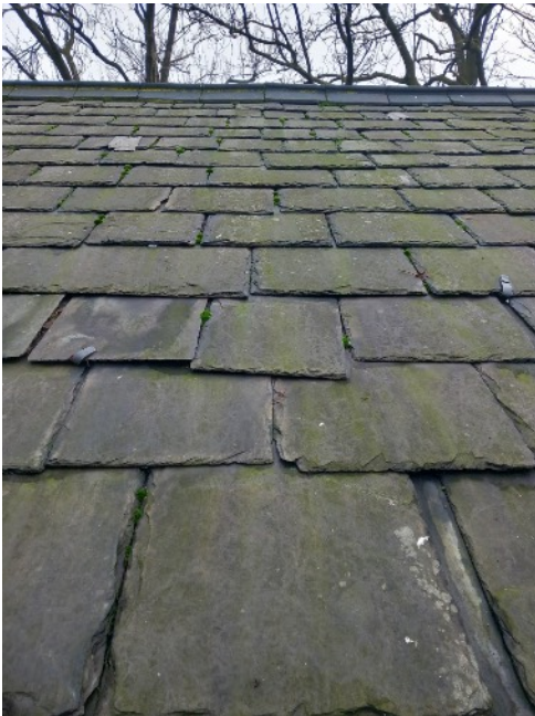
Slates facing front elevation
