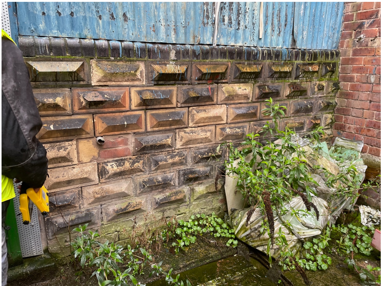
Terracotta Sample Panel (external view), March 2022.
