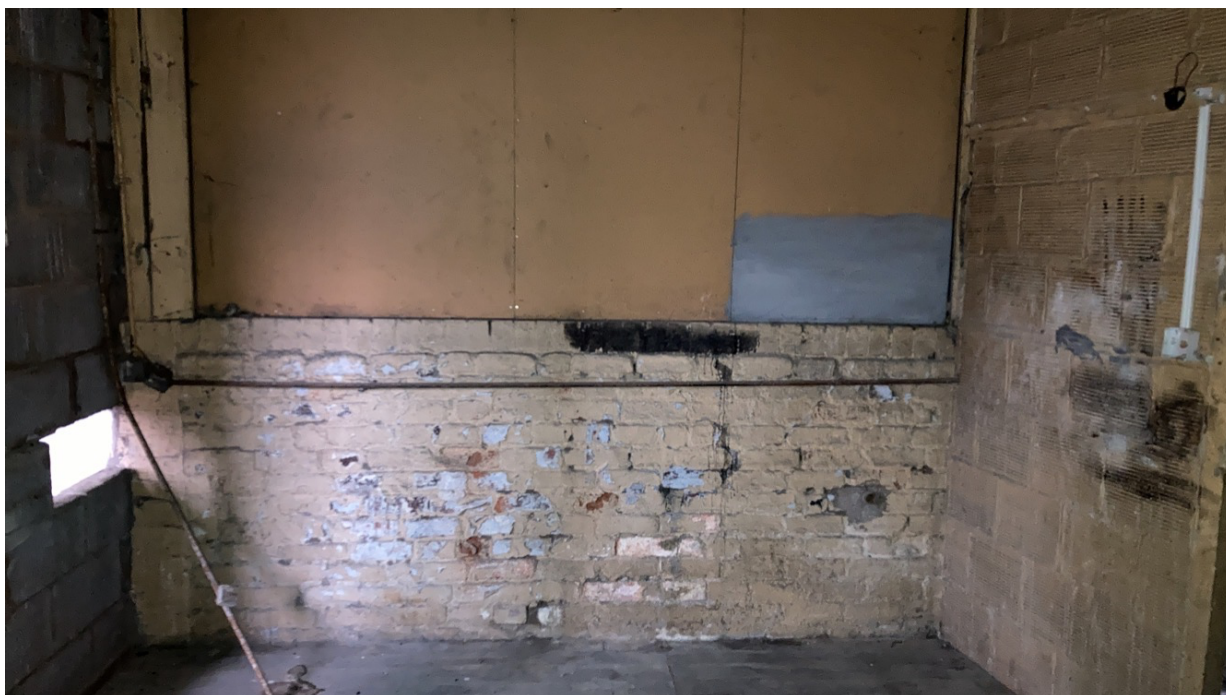
Terracotta Sample Panel (internal view showing brickwork inner face), April 2022.
