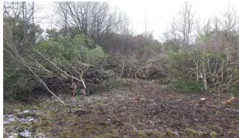
Photograph 3 (P3) Cleared vegetation and overgrown areas in the southwest of the site.
