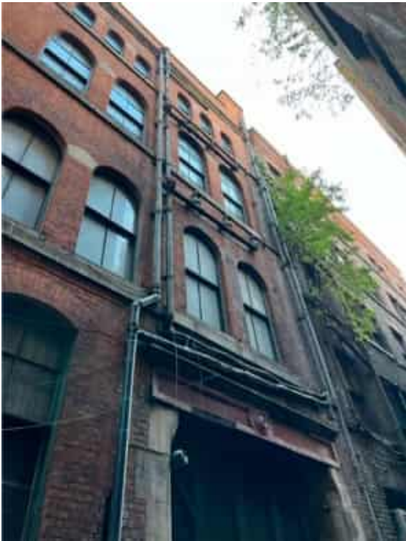
Photo 3, All foul water drainage from upper floor levels is located on the external walls.
