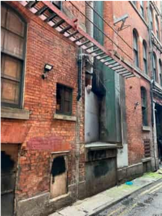
Photo 1, A number of external pipes located to the side of the building, ultimately end up in MH01 and MH02
