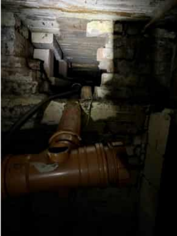
Photo 11, RE1 (rodding point 1) view heading up towards existing toilets
