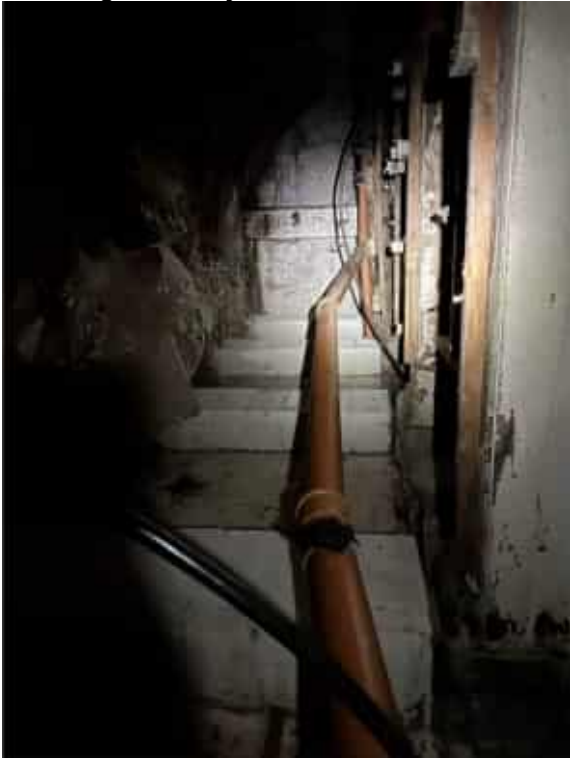
Photo 4, Drainage located in basement - RE1 and RE2 from the CCTV Drainage Survey
