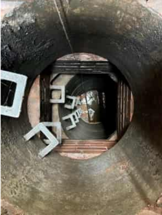
Photo 13, View down public sewer manhole - depth of manhole is 5.18m
