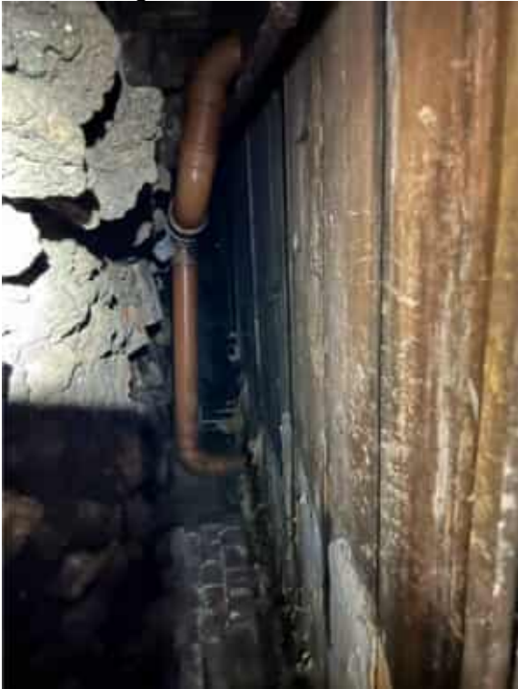
Photo 7, Drainage pipes under the Lower Ground Floor - previously served the existing toilets
