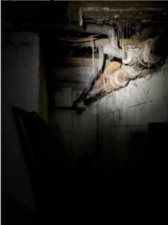
Photo 6, Drainage located in basement - this picture shows the main outfall pipe heading towards MH01
