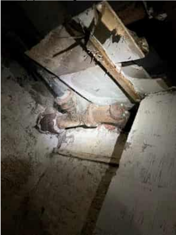
Photo 8, Picture shows the point where the basement sump connects to the main pipe leaving site
