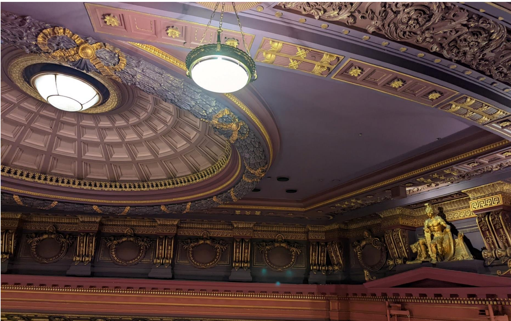
Existing auditorium ceiling services
