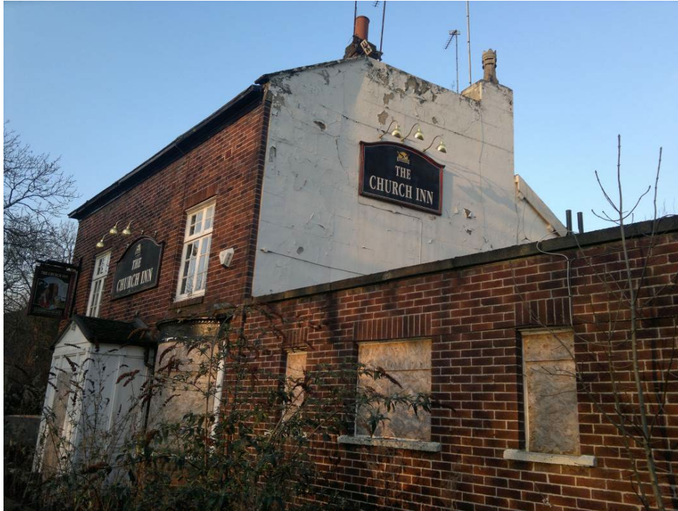
Figure 13: The Inn seen here in 2013 following its closure in c2012.
