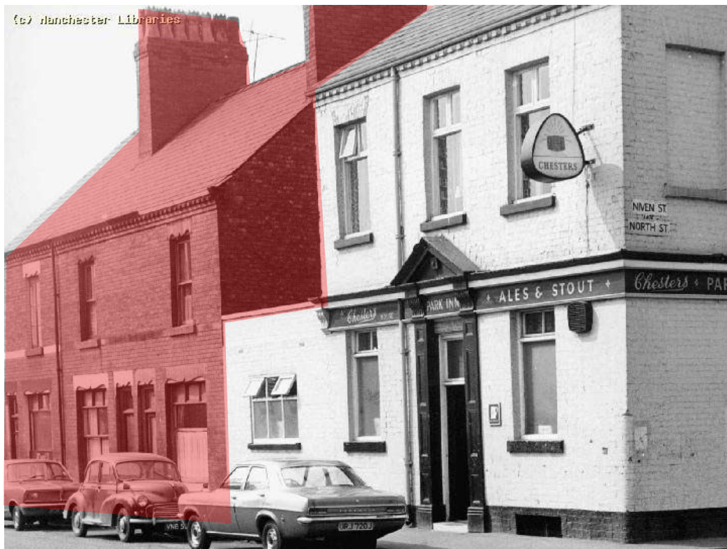
Figure 20: No's 11, 13 and 15 Chapel Street as seen in 1971 (shaded red). Source: Manchester Local Archives.
