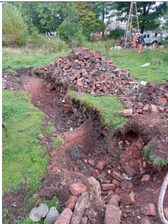
Photo 8: Showing foundation brick wall (left) and paving (right) exposed at the surface around TP07, facing north.
