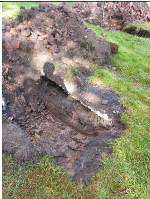
Photo 7: Showing foundation brick wall (right) and paving (left) exposed at the surface around TP05 & TP06, facing north.
