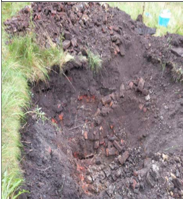
Photo 3: Showing made ground and brick wall in TP04, facing south west.
