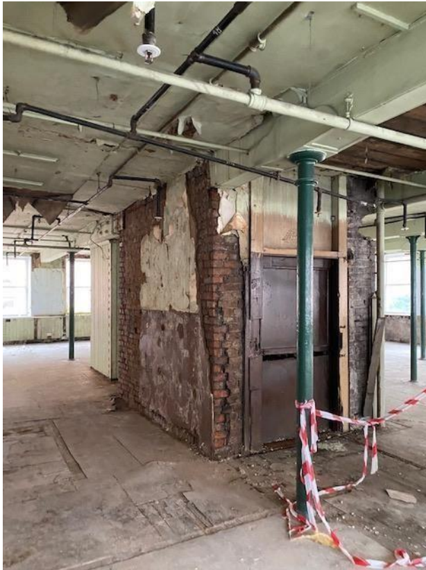
Mindel House Fourth Floor wall lime plaster
