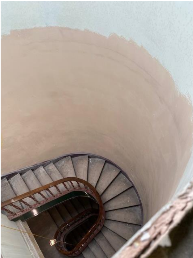
Gypsum plaster enclosing geometric staircase
