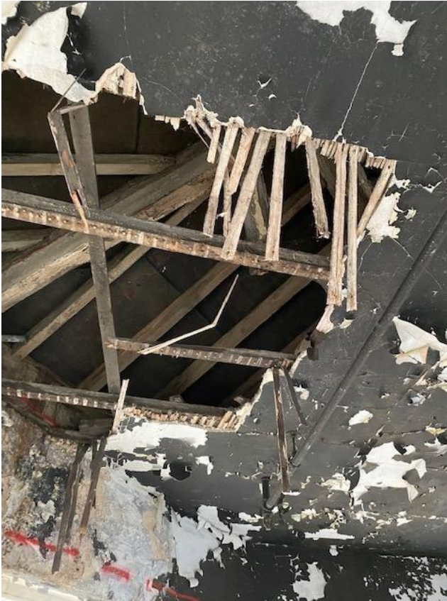
Mindel House Fourth Floor Lath and Plaster Ceiling
