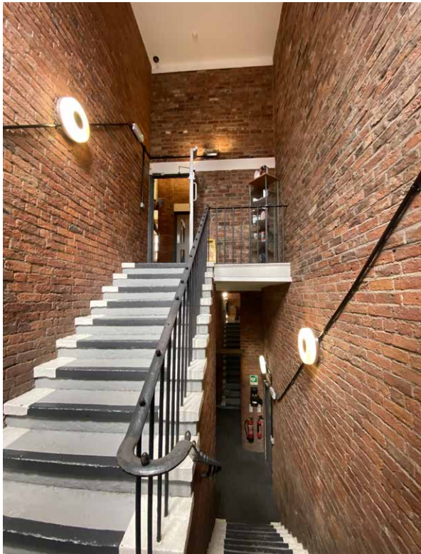
Stone stair to first floor
