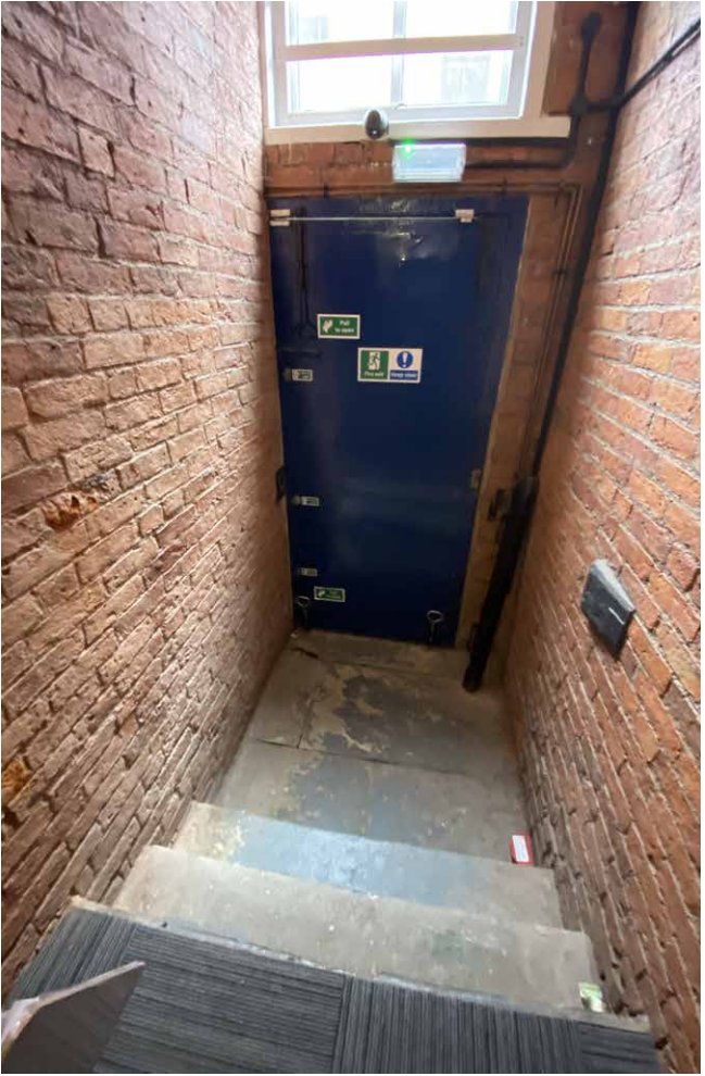
Stepped exit to school street
