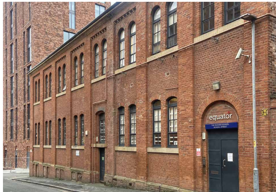
South East elevation, showing entrance on School Street, post 2010 work. New door/signage, windows and sill treatment.
