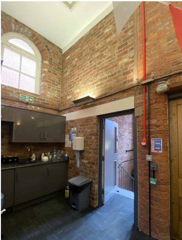
Kitchenette to main first floor corridor, showing modern infill brickwork
