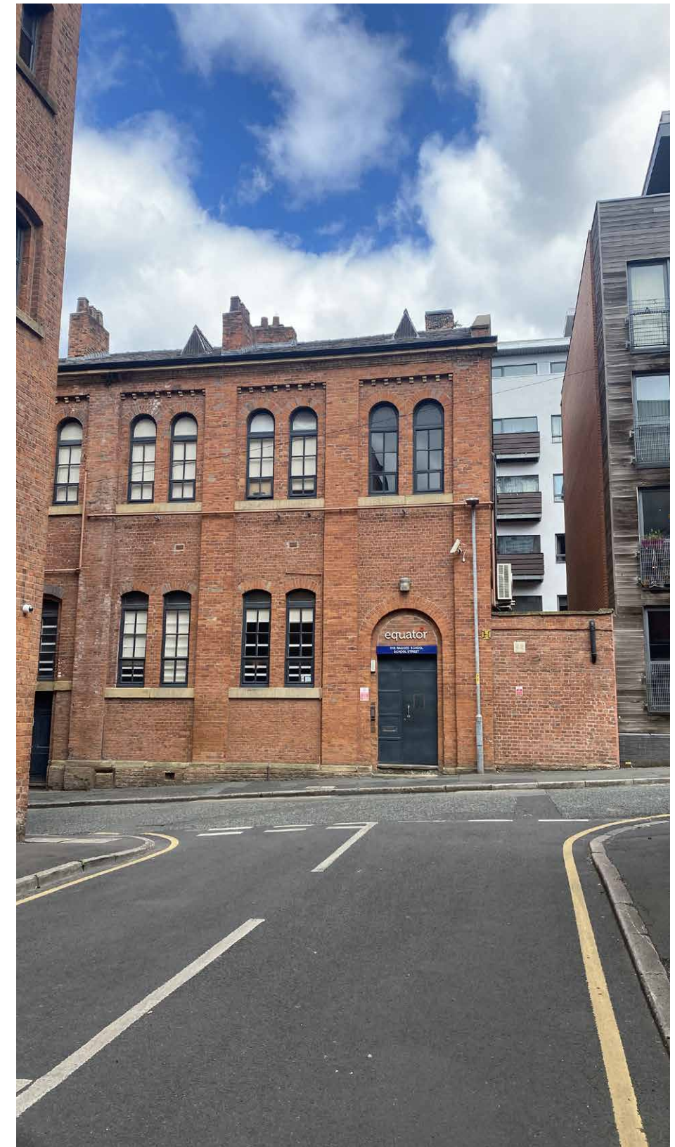
Main Entrance on School Street
