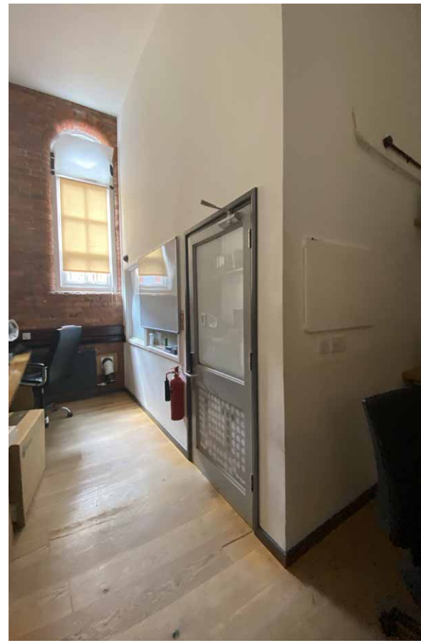
Comms room, modern infill
