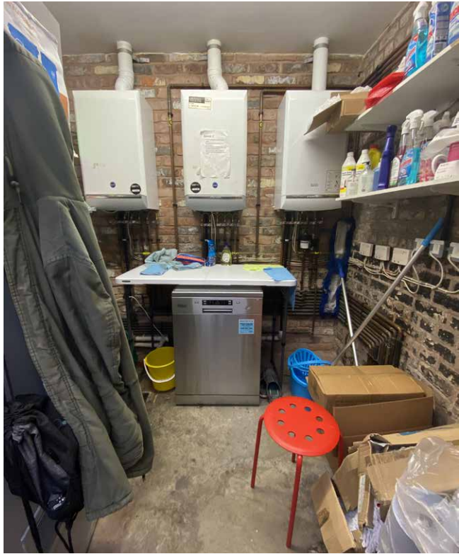
Remodelled boiler room and store
