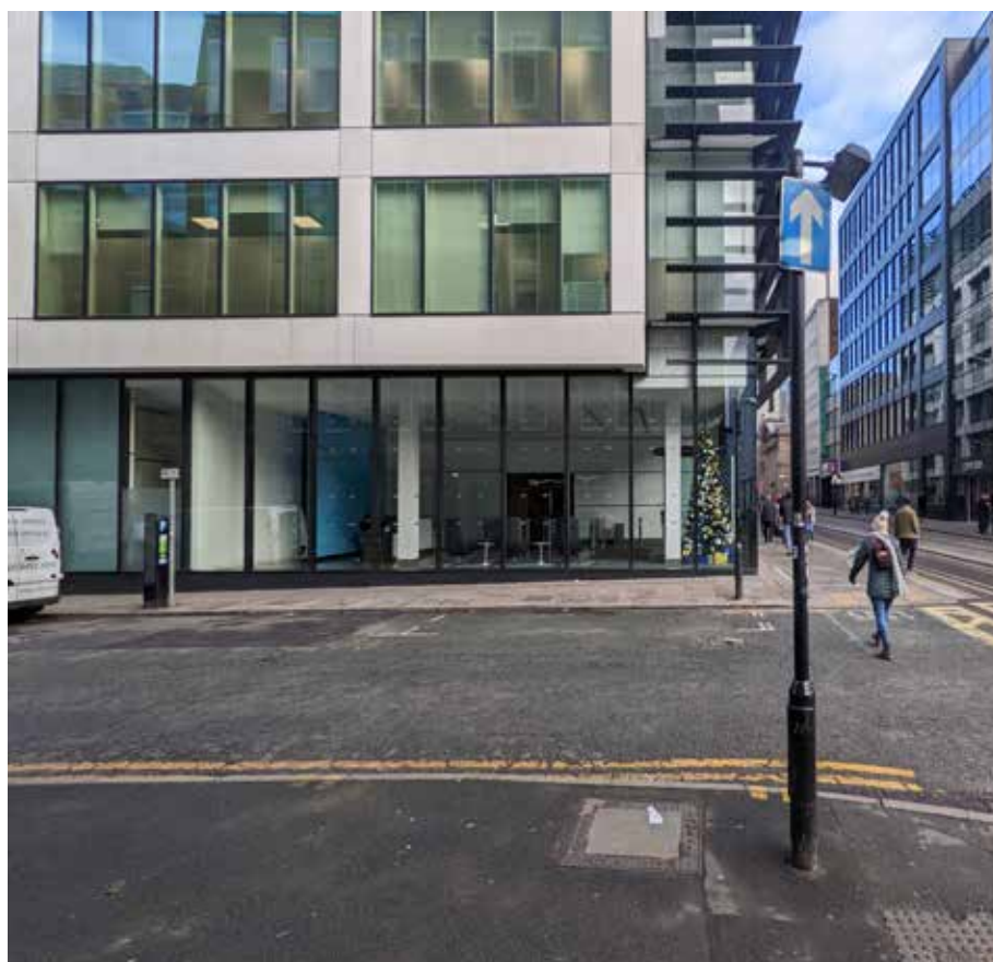
View of reception from Booth Street
