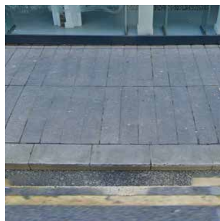
Concrete Slab Paving
