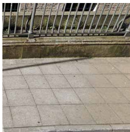
Concrete Slab Paving
