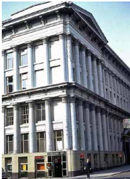
The Milne Building previously occupied the site before being demolished in 1973
