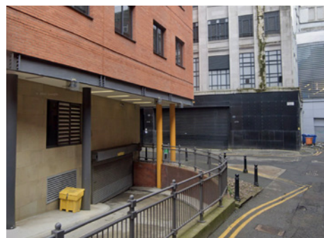
VIEW OF THE BASEMENT ENTRANCE RAMP FROM WEST MOSLEY STREET
