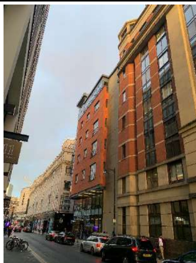
Figure 2 – Looking north east, showing the adjacent building and third party wall (beige column) shared with the building on site.
