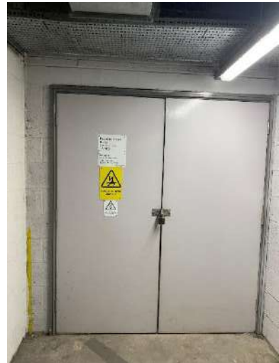
Figure 10 – Looking west, showing the outside of the electricity sub station.
