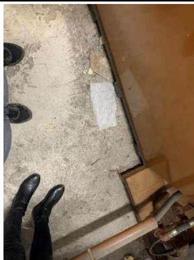
Figure 6 – Showingno evidence of spills or leaks on the floor around the diesel tank.
