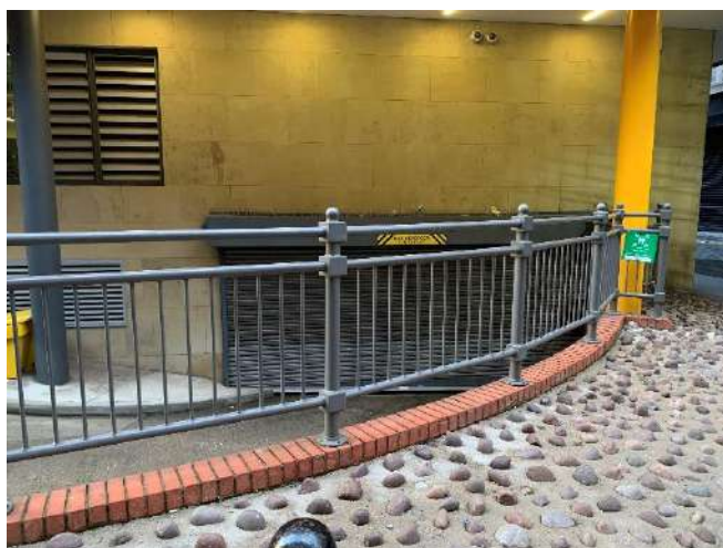
Figure 3 – Looking west, showing the entrance to the basement carpark from West Moseley Street.
