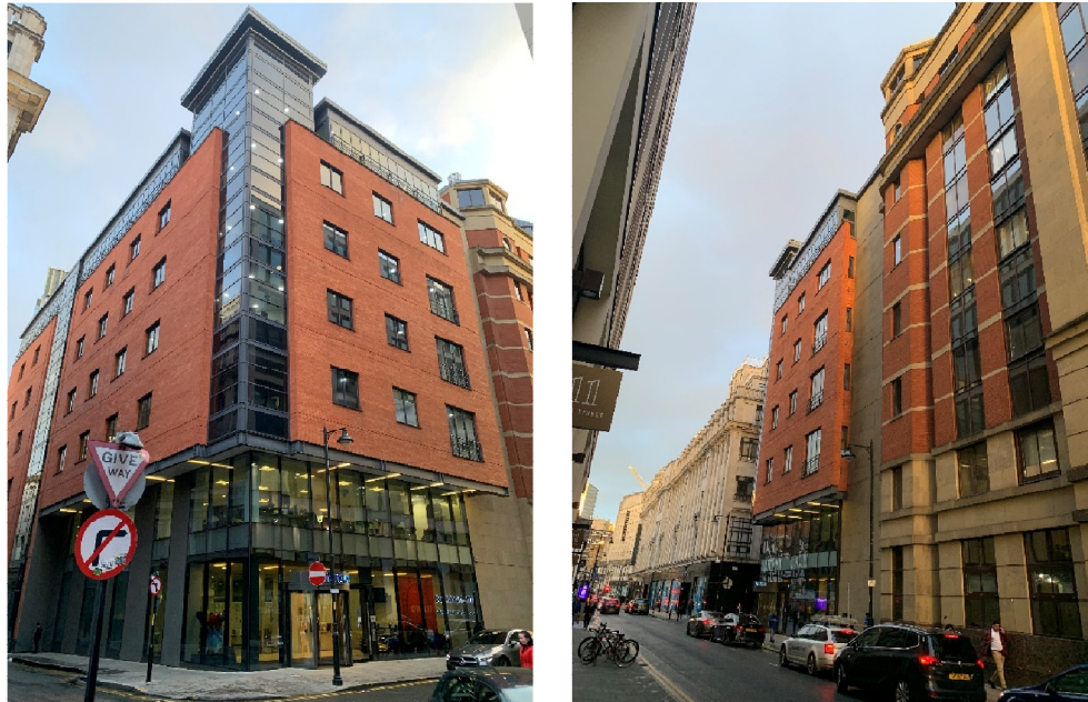
Figure 2: Photographs of the existing building, showing the main entrance, looking southeast (left) and from the south, showing the third party wall (beige column), looking northeast (right).
