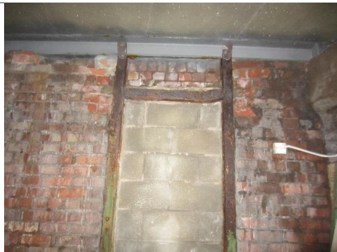
Photo 20: Well-pointed brick walls and steel roof at off-site stores beneath New Quay Street
