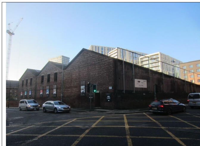
Photo 1: South-eastern and north-eastern elevations of the Shipyard building
