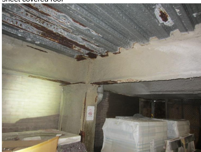
Photo 18: Steel and concrete at the ceiling of the undercroft
