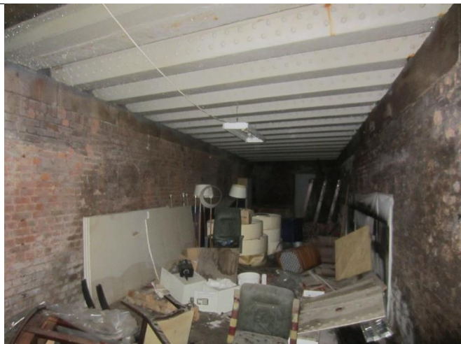
Photo 19: Well pointed brick walls and steel roof at off-site stores beneath New Quay Street
