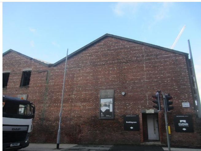
Photo 4: South-eastern elevation at Water Street
