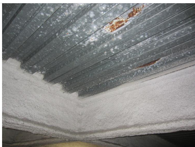
Photo 17: Steel and concrete at the ceiling of the undercroft
