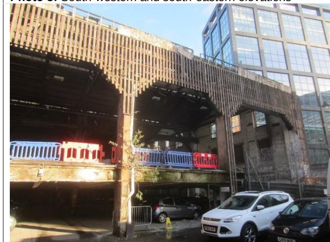
Photo 5: South-eastern elevation showing street level and undercroft
