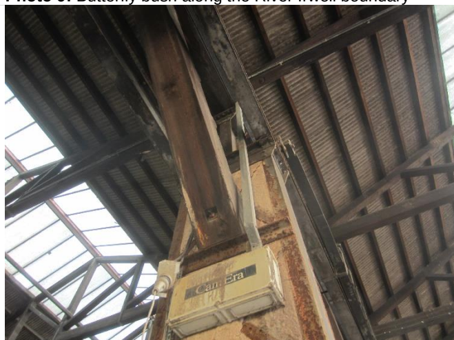
Photo 11: Steel and timber frame supporting corrugated sheet covered roof
