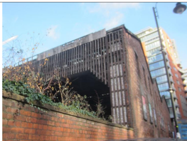
Photo 2: South-eastern elevation at Water Street
