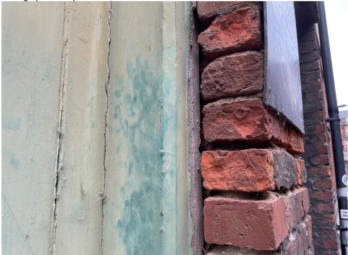
Photograph 4 – Gaps surrounding the loading bay.
