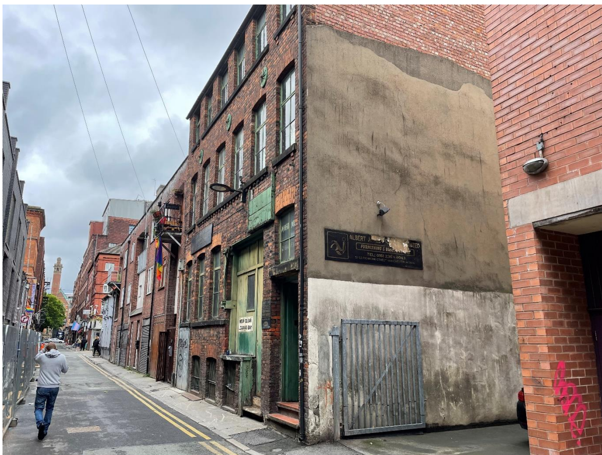
Photograph 1 – The north-west corner of 51-53 Richmond Street.
