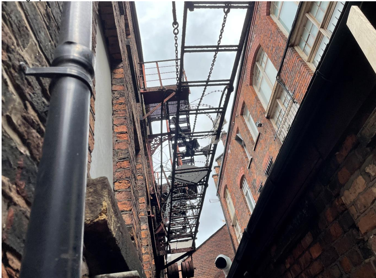
Photograph 2 – The south-east facing rear of the building.
