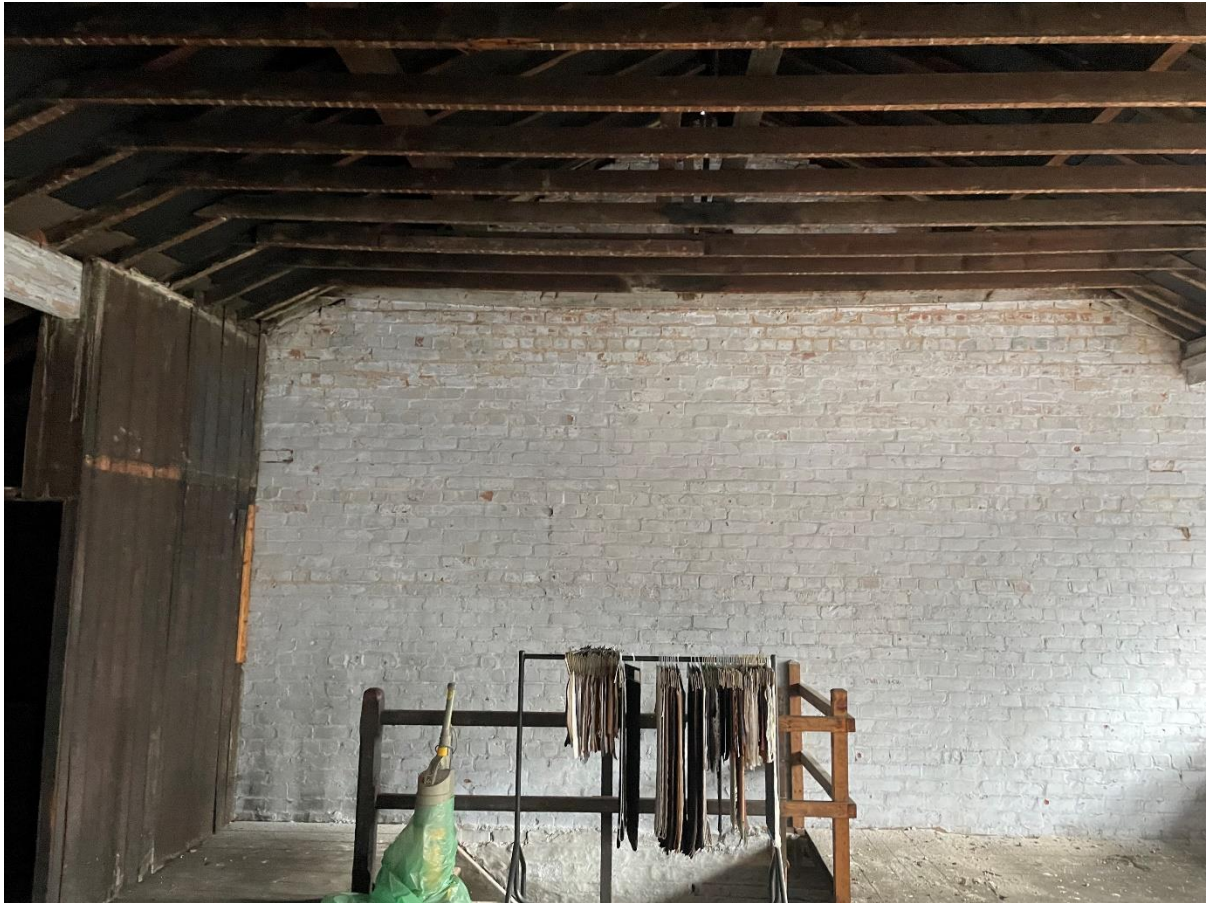
Photograph 7 – Internal south-west aspect.
