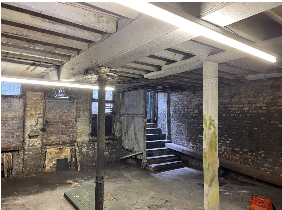
Photograph 15 – The north-eastern corner of the cellar.
