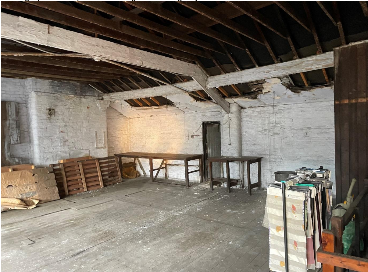
Photograph 6 – Internal eastern facing corner.
