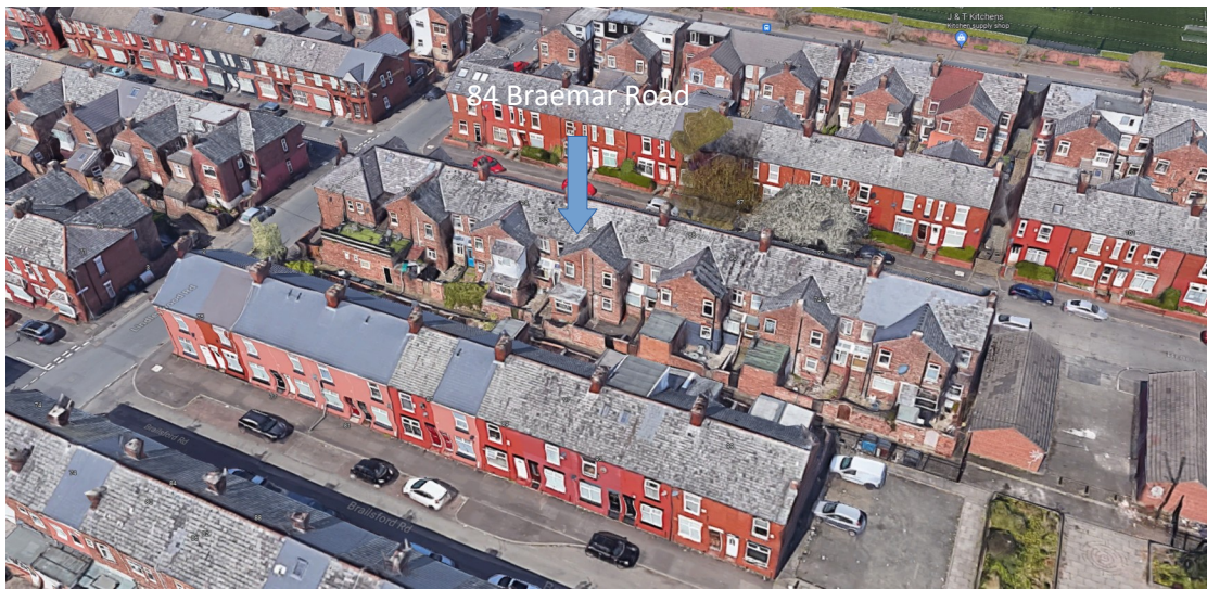
Aerial view courtesy of Google Earth
