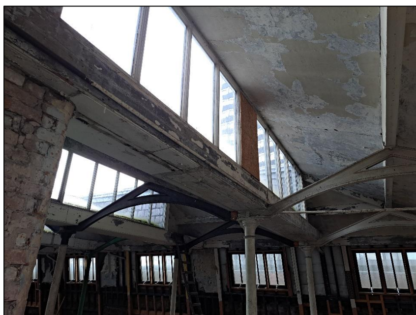
Photograph 6 showing the skylights and windows of the upper floor
