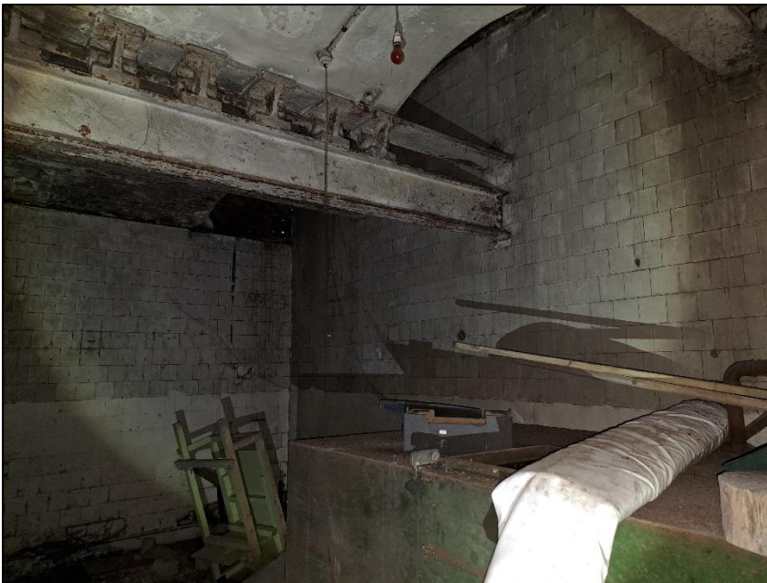
Photograph 18 showing one of the basement rooms
