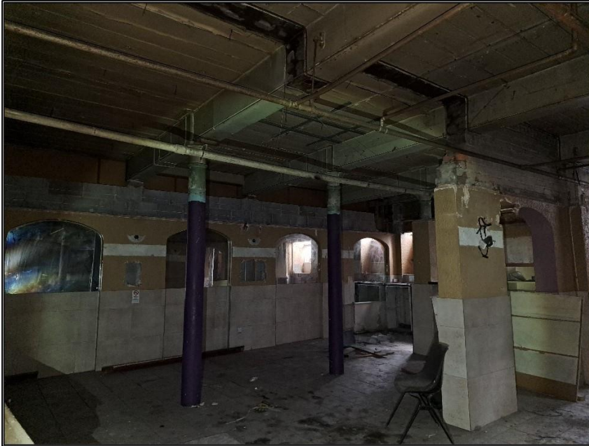
Photograph 17 showing one of the basement rooms
