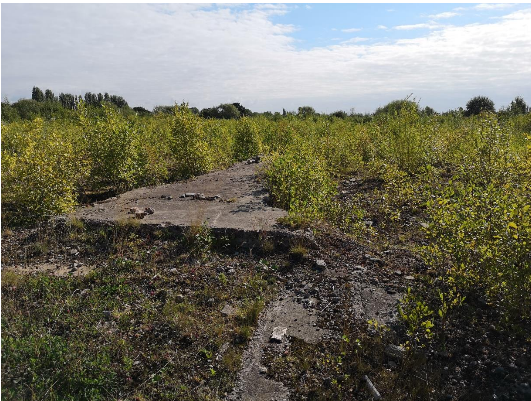
Plate 4 View of foundations toward the southern boundary, looking east
