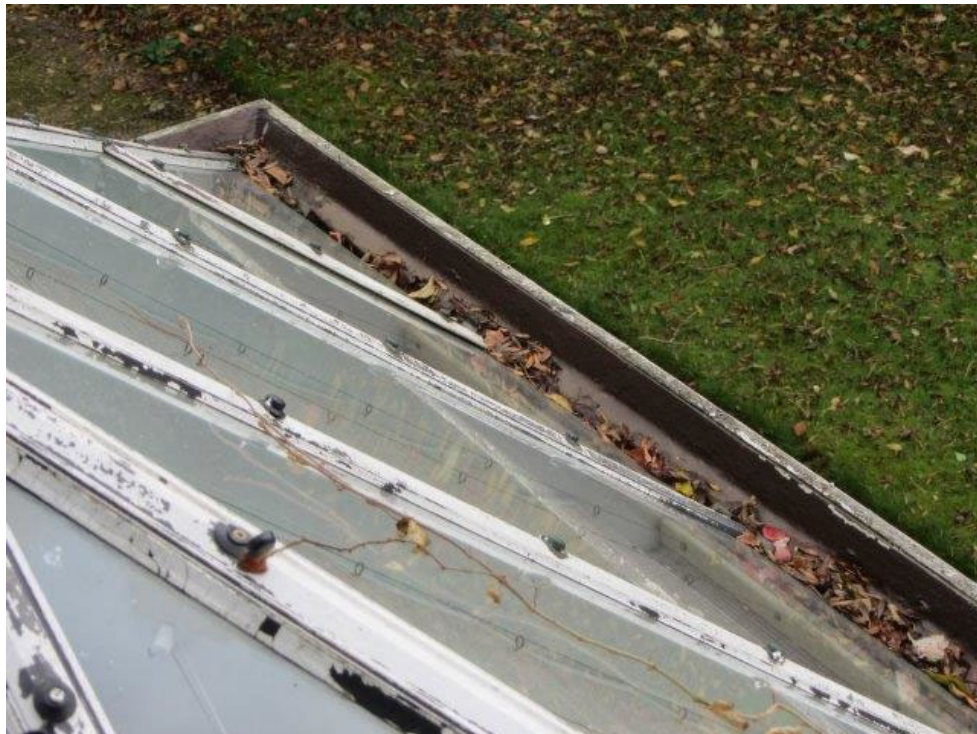
Image 19: Timber faced fibreglass gutters to perimeter
