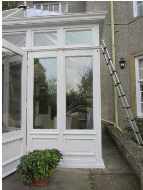
Image 4: Bowing to corner post
