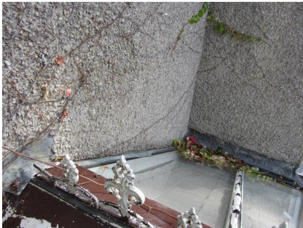
Image 14: Low dressed lead flashings at abutment to main building
