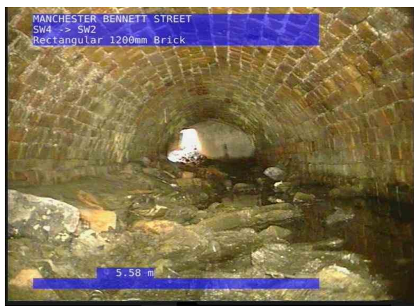
SW2X_a88a306d-51f2-4a36-a121-17afa1dd8b30_20220715_100125_460.jpg, 00:00:53, 5.58 m General photograph taken at this point
