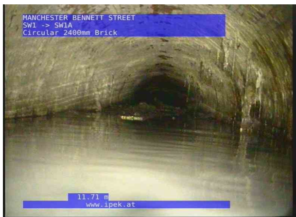
SW1AX_9e94d0b0-ae5c-4be1-9cb5-7a6e0b762e7f_20220715_115443_829.jpg, 00:02:22, 11.71 m General photograph taken at this point
