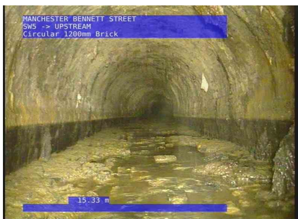
UPSTREAMX_54fd5ad1-e941-401a-bc7d-19417c17db05_202 20715_102522_812.jpg, 00:05:07, 15.33 m General photograph taken at this point
