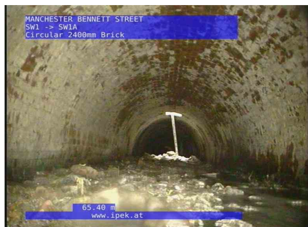
SW1AX_159c681b-d58a-44f0-80ac-01975f994ab5_20220715_120628_265.jpg, 00:13:40, 65.40 m General photograph taken at this point
