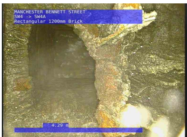
SW4X_f82995f1-0c30-4031-b276-b723afe879cc_20220714_1 00152_117.jpg, 00:00:44, 4.29 m Finish node, manhole, reference: SW4A
