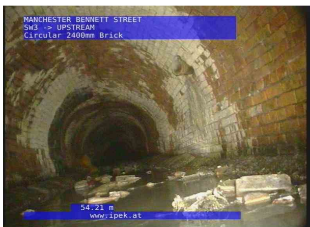
UPSTREAMX_0b485ba5-5288-470d-80f6-2e5df68dc5cb_202 20715_122500_711.jpg, 00:05:40, 54.21 m Finish node, other special chamber, reference: UPSTREAM, SITE BOUNDARY
