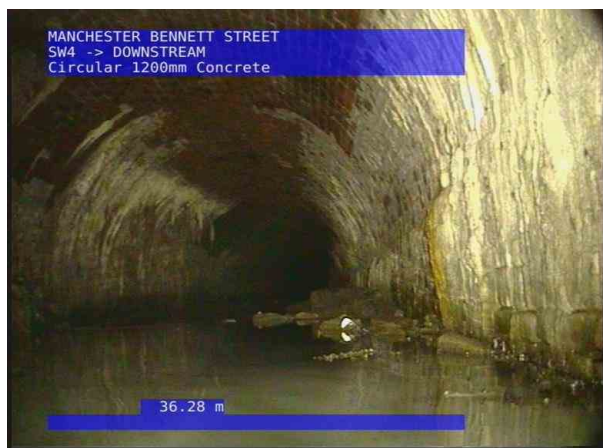
SW4X_cc0334c9-a616-4d7a-b5a4-fc2cd2ed6b95_20220715_110755_523.jpg, 00:08:28, 36.28 m Finish node, other special chamber, reference: DOWNSTREAM, DOWNSTREAM
