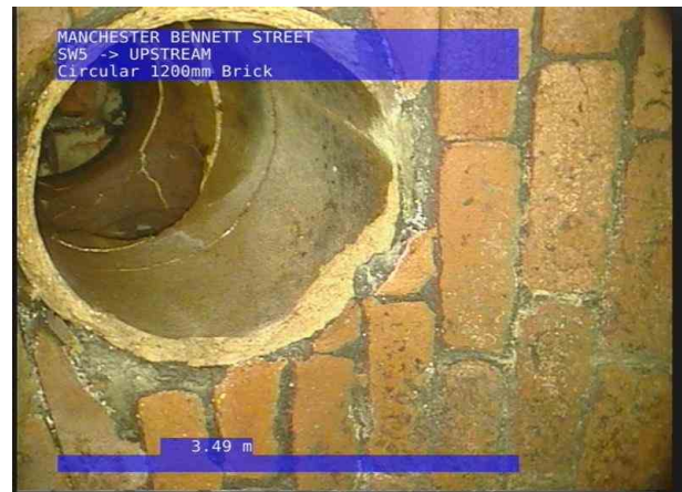
UPSTREAMX_dcff5fe2-aeff-490b-995b-ba493665b4b6_20220 715_102025_082.jpg, 00:00:29, 3.49 m Connection other than junction at 10 o'clock, 150mm dia
