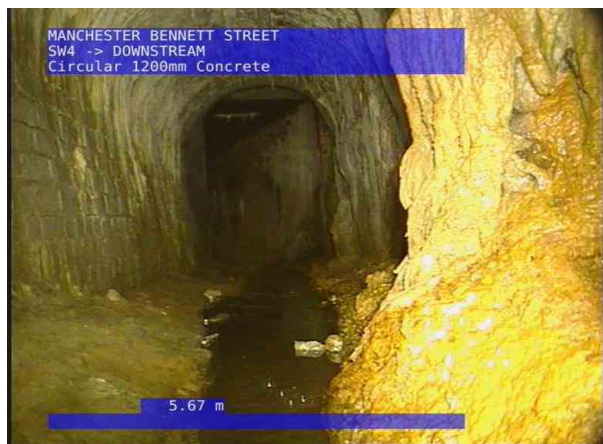
SW4X_7ba24df5-5b44-43ee-a792-b98ed0a69942_20220715_110051_763.jpg, 00:01:40, 5.67 m General photograph taken at this point
