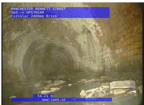
UPSTREAMX_dfbf69c7-bc0a-4c33-b12f-5eabe869bd7c_2022 0715_122414_593.jpg, 00:05:15, 54.21 m General photograph taken at this point
