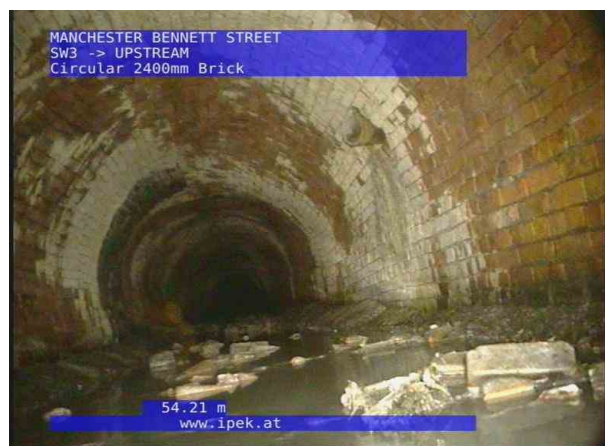
UPSTREAMX_991564bf-0861-4d4b-a1df-d86103db70fa_202 20715_122425_384.jpg, 00:05:16, 54.21 m Connection other than junction at 2 o'clock, 150mm dia
