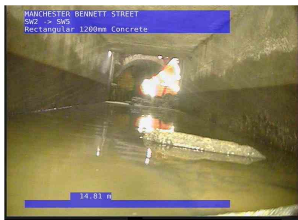
SW5X_ac348325-cd20-46ec-826f-070bdde3b9d5_20220715_101353_898.jpg, 00:04:03, 14.81 m General photograph taken at this point
