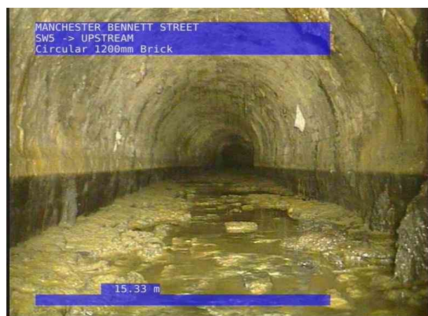
UPSTREAMX_116c7368-fcb8-46bb-ac8c-c52e9c534ca7_202 20715_102632_146.jpg, 00:05:53, 15.33 m Settled deposits, fine, 10% cross-sectional area loss
