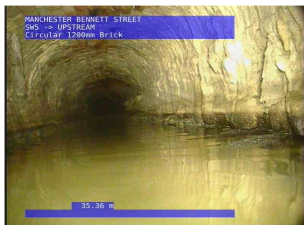
UPSTREAMX_377dde82-9c8f-4f1f-a704-8ae6e5bb81a1_2020715_103244_452.jpg, 00:11:50, 35.36 m General photograph taken at this point
