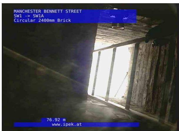
SW1AX_9850a96d-4115-417e-8810-21b0ce4ed79d_20220715_120924_196.jpg, 00:16:25, 76.92 m Finish node, manhole, reference: SW1A
