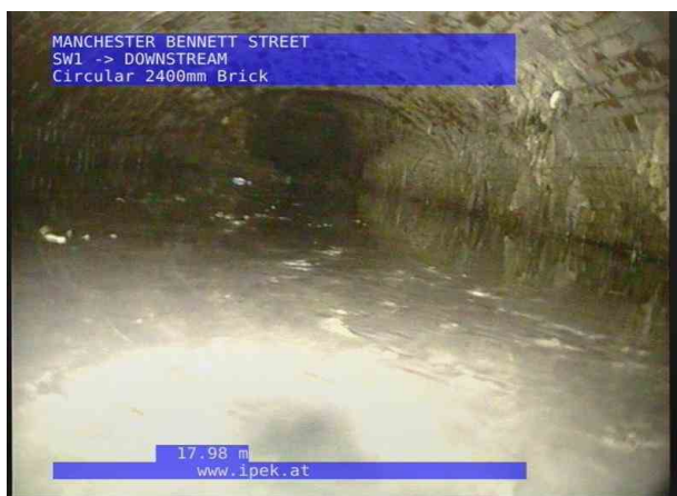
SW1X_636893ad-f8cd-40c8-821c-0b3c21f6783e_20220715_114156_760.jpg, 00:11:46, 17.98 m General photograph taken at this point
