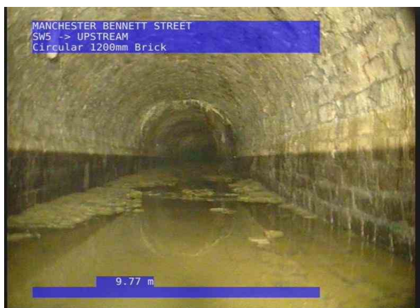
UPSTREAMX_3ed8743e-5dce-4b7d-87ee-8c3bde5c8864_20 220715_102215_180.jpg, 00:02:03, 9.77 m General photograph taken at this point
