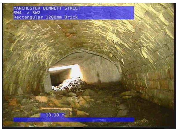
SW2X_758cbab1-3929-4c78-9e62-1d542afddf8b_20220715_100531_529.jpg, 00:03:30, 10.10 m General photograph taken at this point
