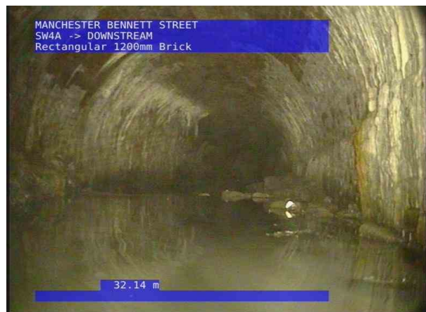
SW4AX_0de353f5-b381-4786-9876-cd161d4f69a8_20220714_101113_509.jpg, 00:06:31, 32.14 m Finish node, other special chamber, reference: DOWNSTREAM, MEETS UP WITH THE D/S FROM MH SW01
