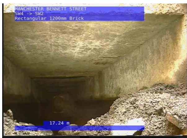
SW2X_03b77516-945e-4afe-8fc8-261587b59a41_20220715_100736_650.jpg, 00:05:23, 17.24 m Finish node, manhole, reference: SW2
