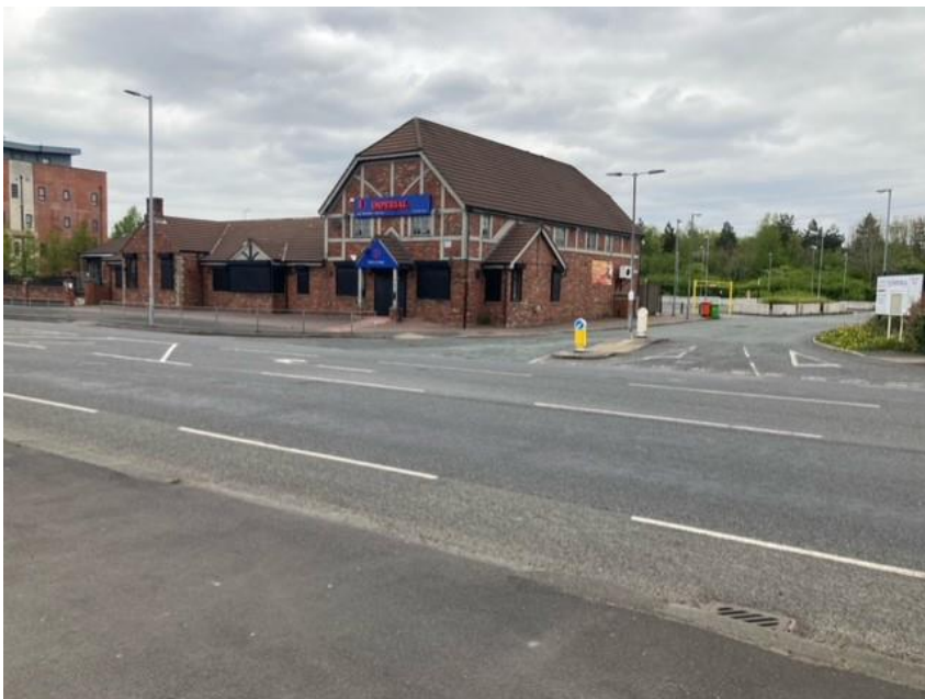
View of existing site as undeveloped
