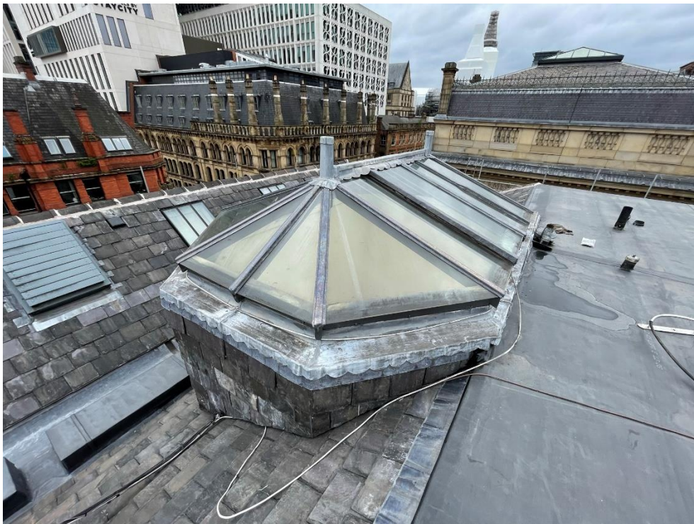
Slated sides to lightwell and leading to rooflight supports
