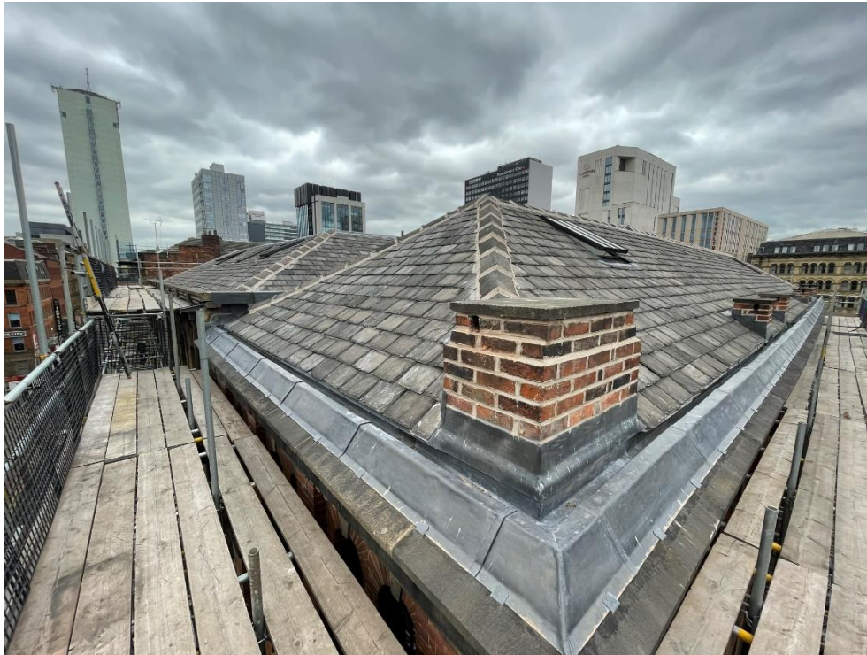
Junction of George Street and Princess Street
