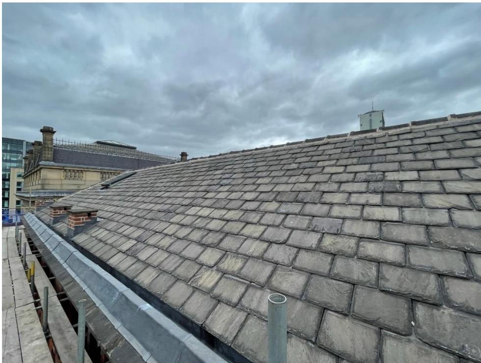
Slate covering to front roof pitch
