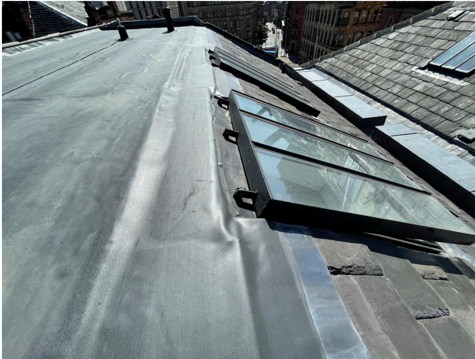
EPDM flat roof dressed onto conservation rooflight flashing
