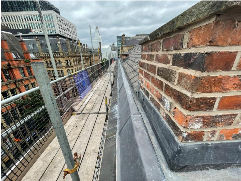
Lead gutter to front elevation
