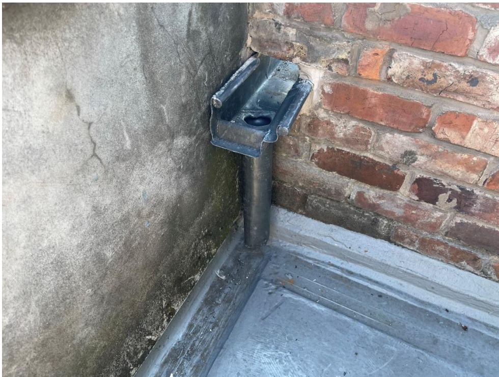
Lead gutter detail onto terrace roof
