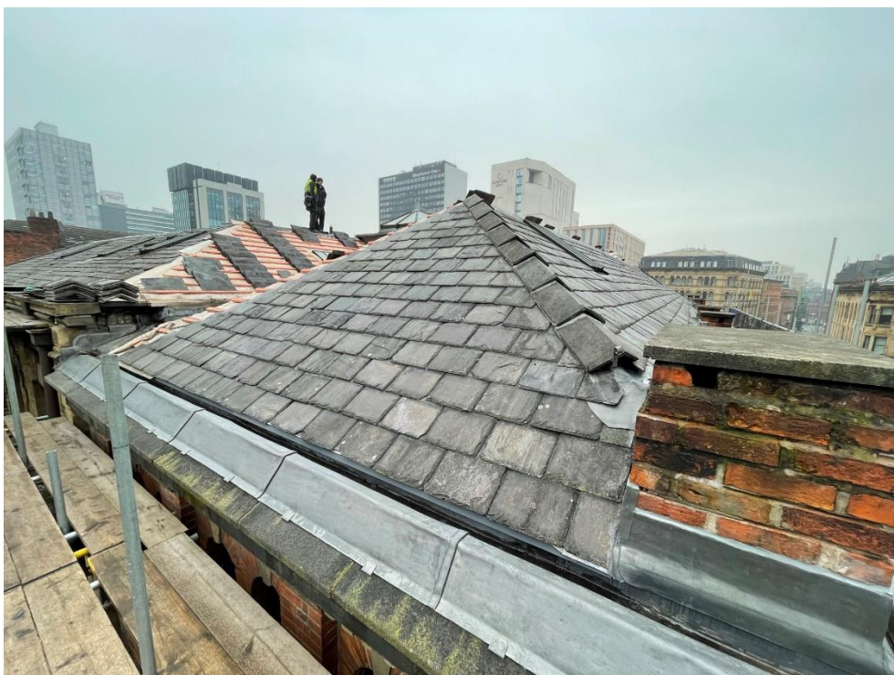
Lead lining to the George Street elevation gutter
