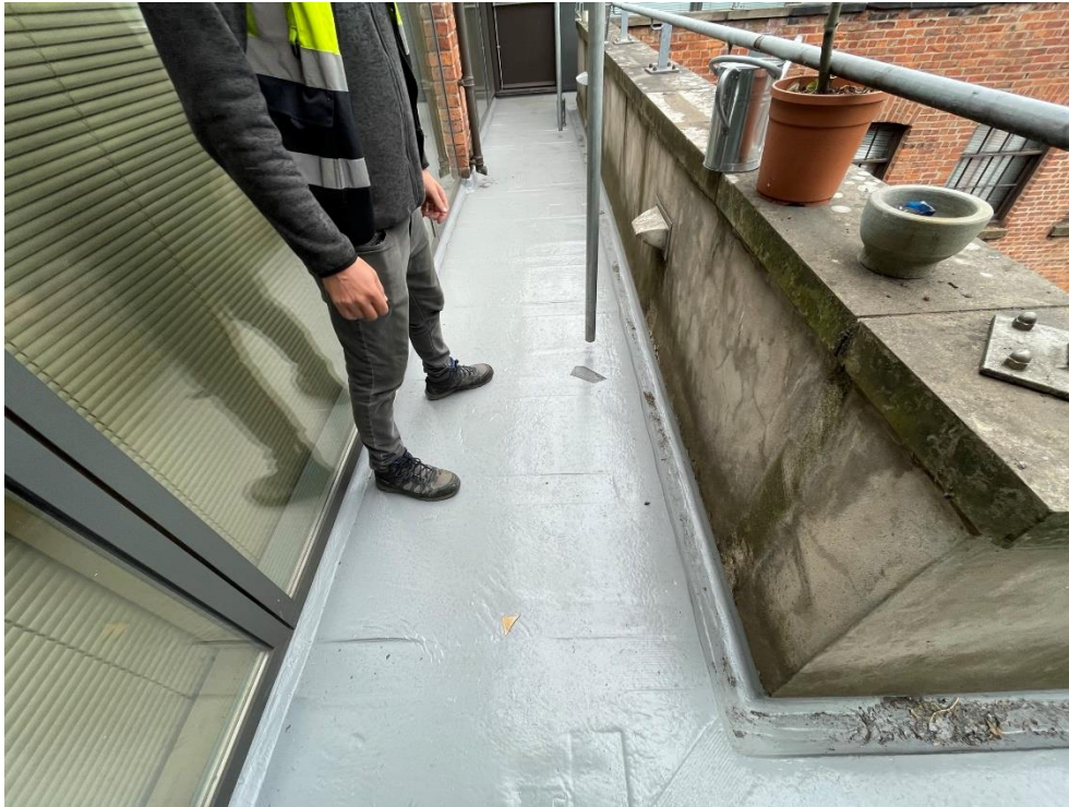
Liquid applied coating to terrace roof, awaiting installation of porcelain tiled finish
