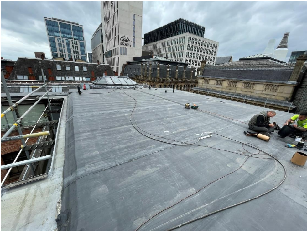
Main flat roof
