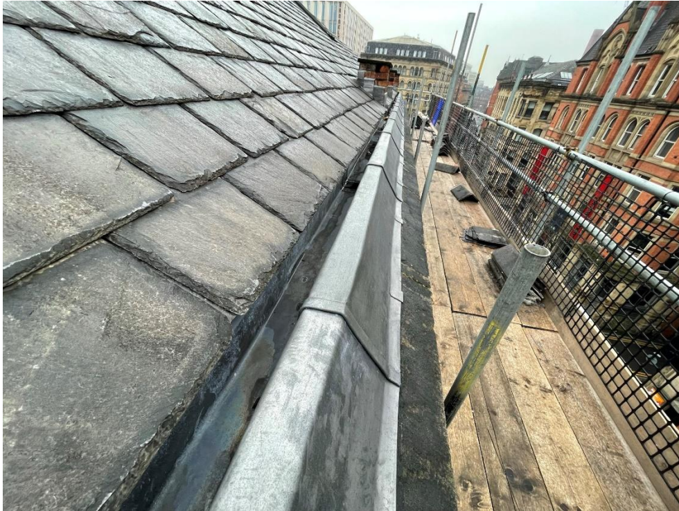
Lead gutter lining to the front elevation.
