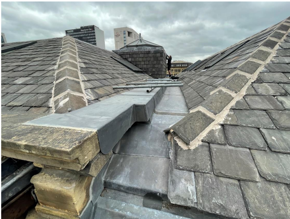
Lead lining to central valley
