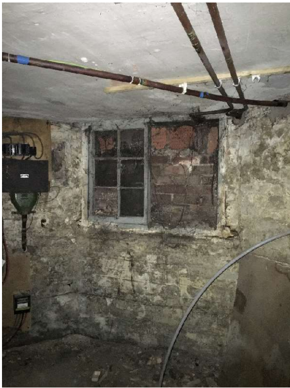
Figure 6.3. Existing basement front window (internal view)
