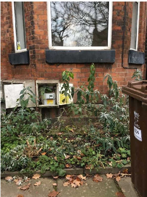
Figure 6.5. Existing basement front window
