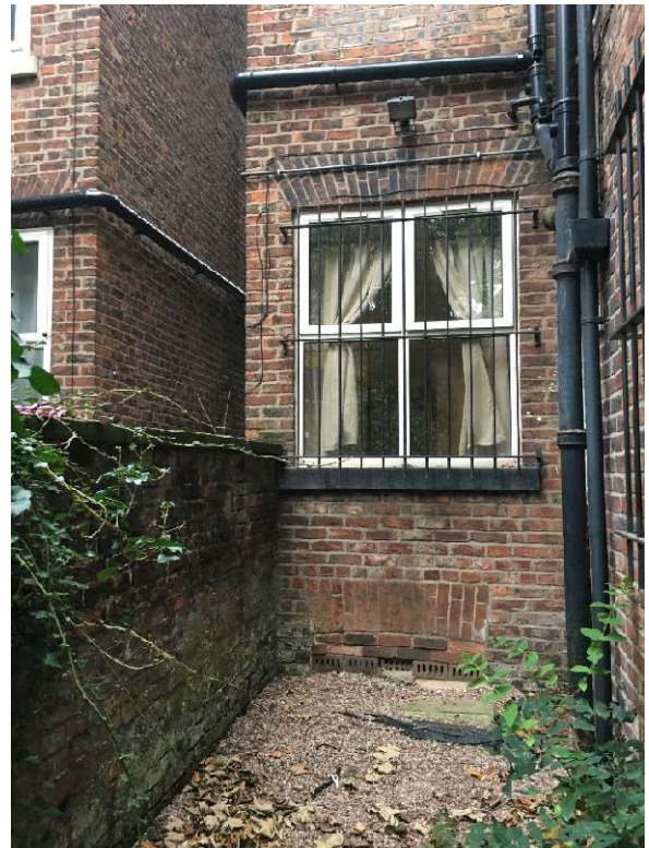
Figure 6.6. Existing basement rear window
