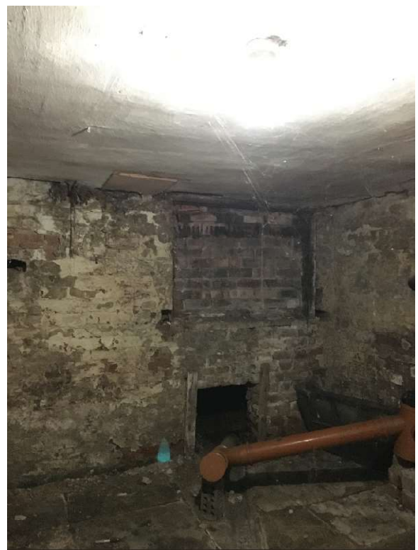
Figure 6.4. Existing basement rear window (internal view)
