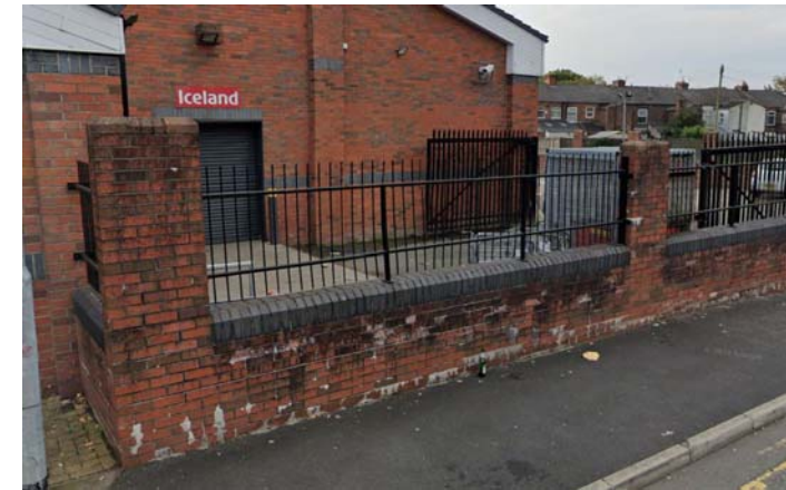
NEIGHBOUR'S PROPERTY BOUNDARY WALL
