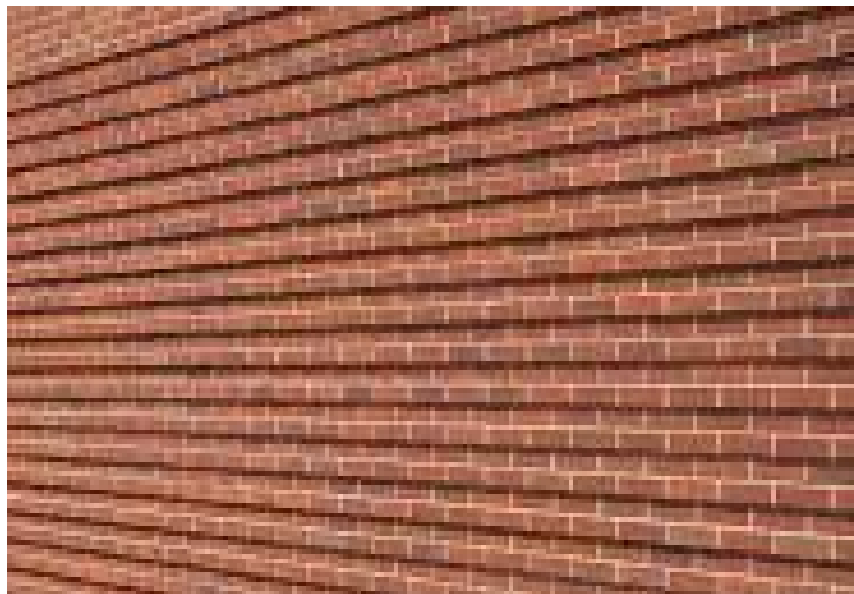
Red Brickwork Detailing
