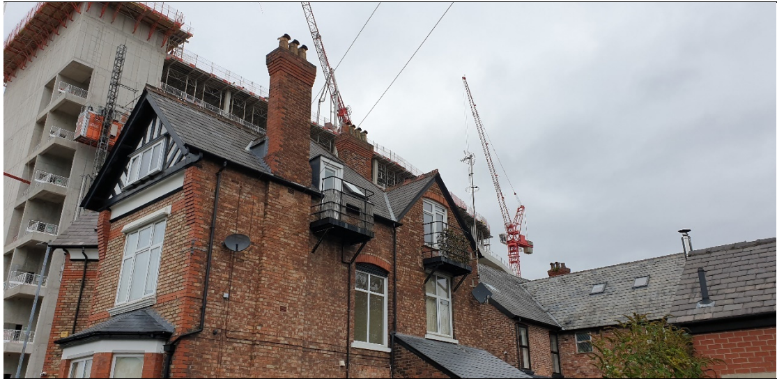
Image 2 – Taken from Rathen Road towards the Site. A close up of the installed antenna showing a communal antenna system with a VHF radio antenna, a DAB radio antenna, a UHF television antenna and a digital satellite television dish present
