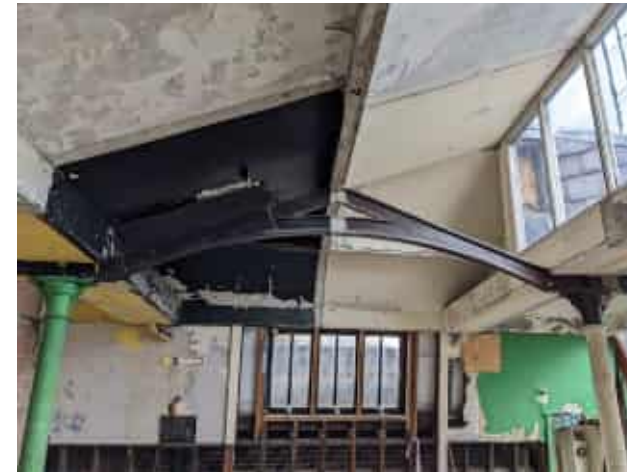
Figure 4 Typical view of internal roof structure.
