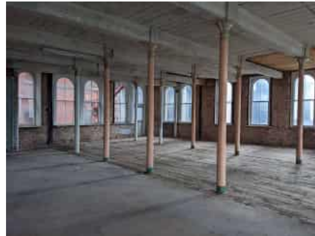
Figure 3 Typical view of upper floors.
