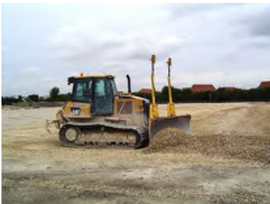
Laser-guided grading of a pitch
