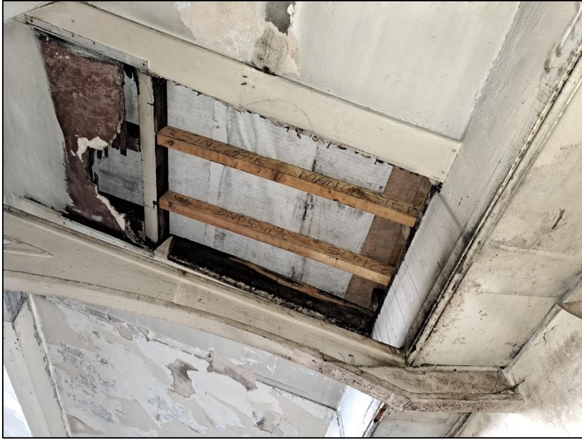
Photograph 9 showing the roof void of the hipped roof
