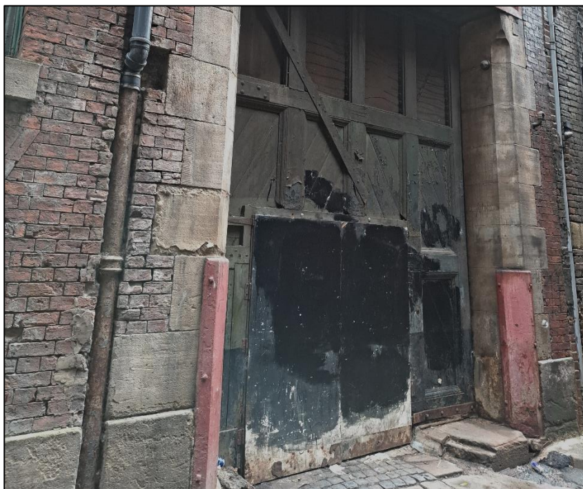
Photograph 2 showing condition of the external brickwork
