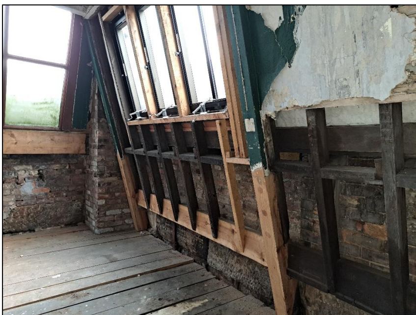
Photograph 5 showing replaced beams
