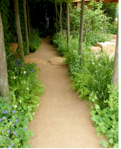
Self binding gravel surface
